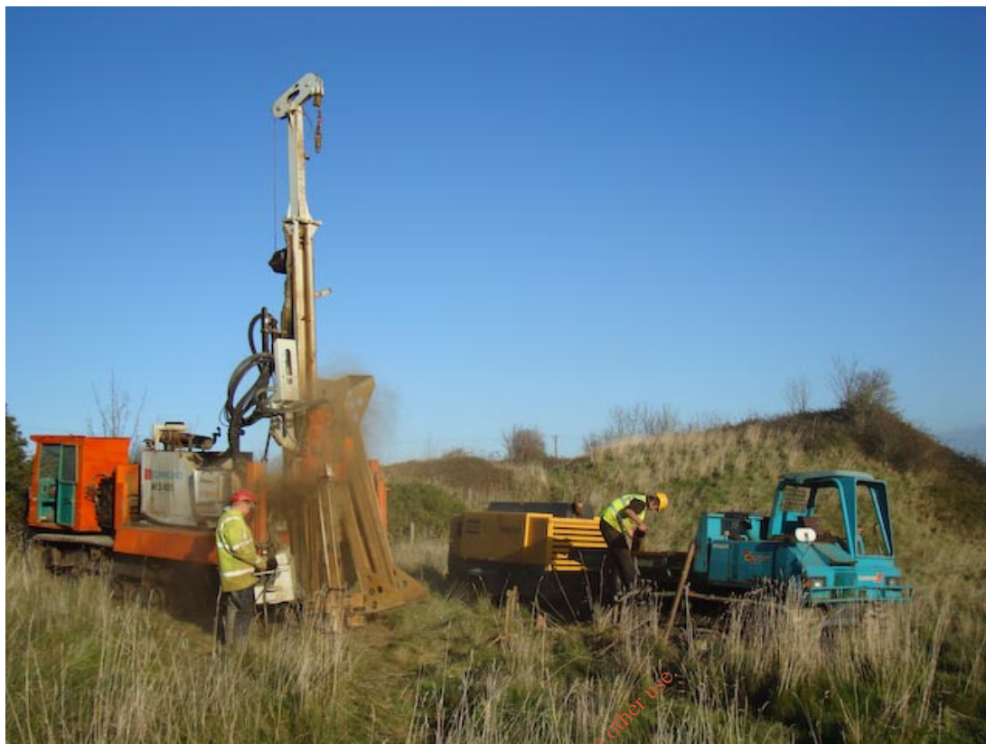
PLATE 6.3 Installation of Groundwater Monitoring Well BH1
