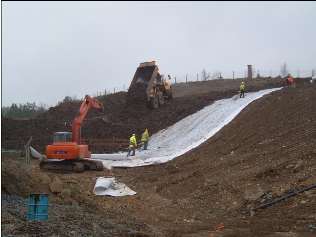
Figure 3: Covering of GCL and geocomposites with subsoil
