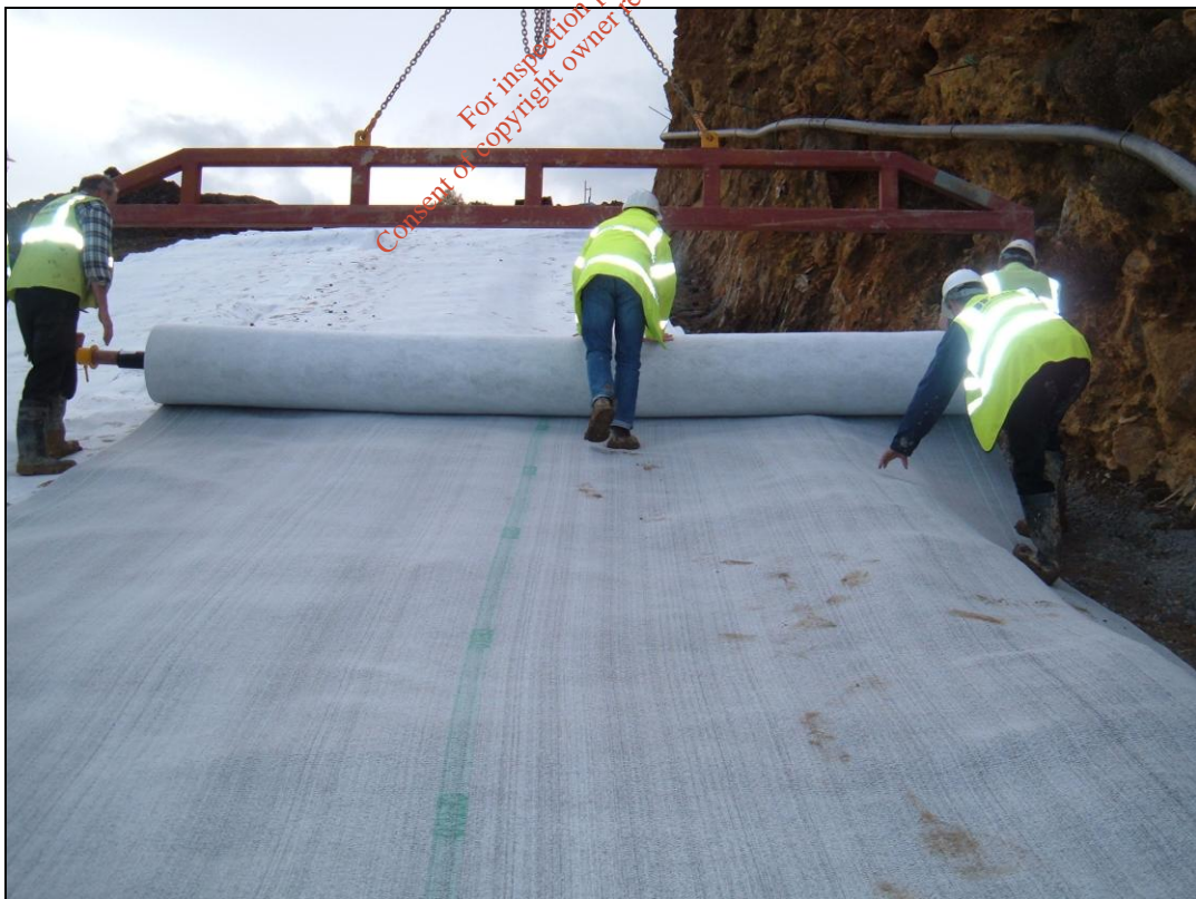
Figure 2: Placement of GCL on top of geocomposite gas collection layer
