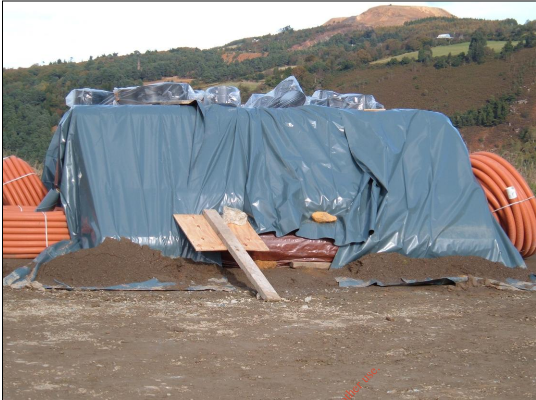
Figure 1: Onsite storage of GCL
