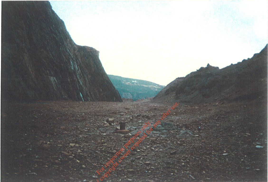
Plate No.8 : East looking view from inside the Ballymurtagh Open Pit.
