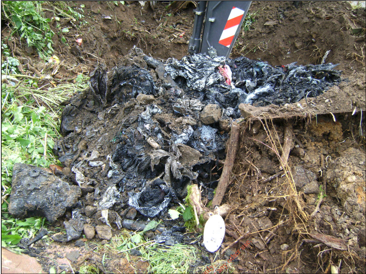
Photo 6 Waste in TP-10
