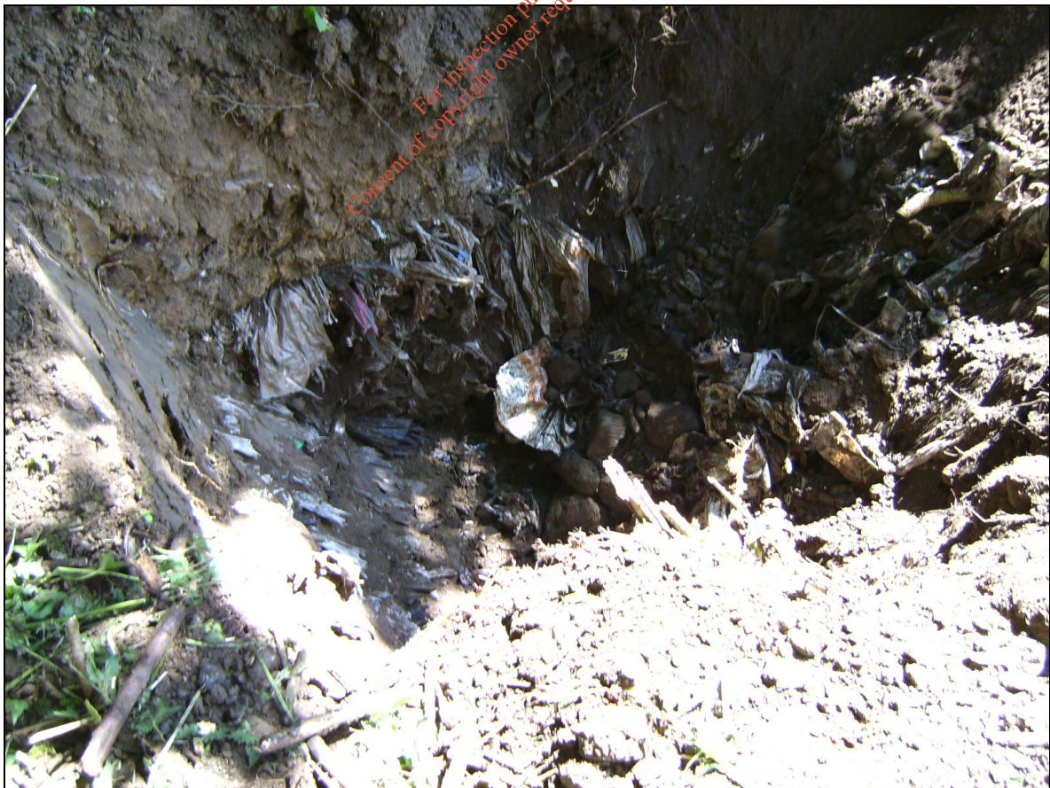
Photo 5 Waste in TP-11
