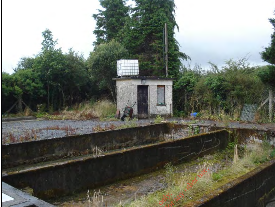
Image 3.3: Pump House and Tanks
