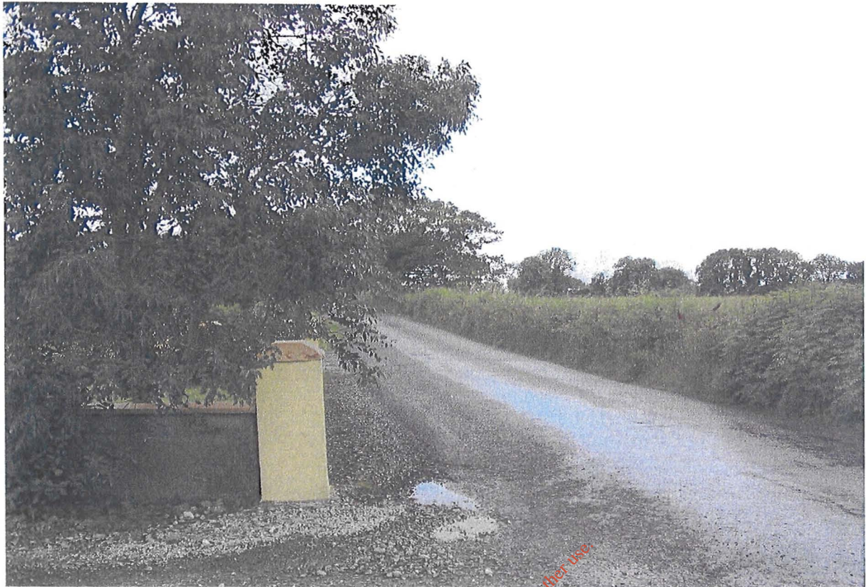
Figure 1.5 Junction at access road to site, looking left
