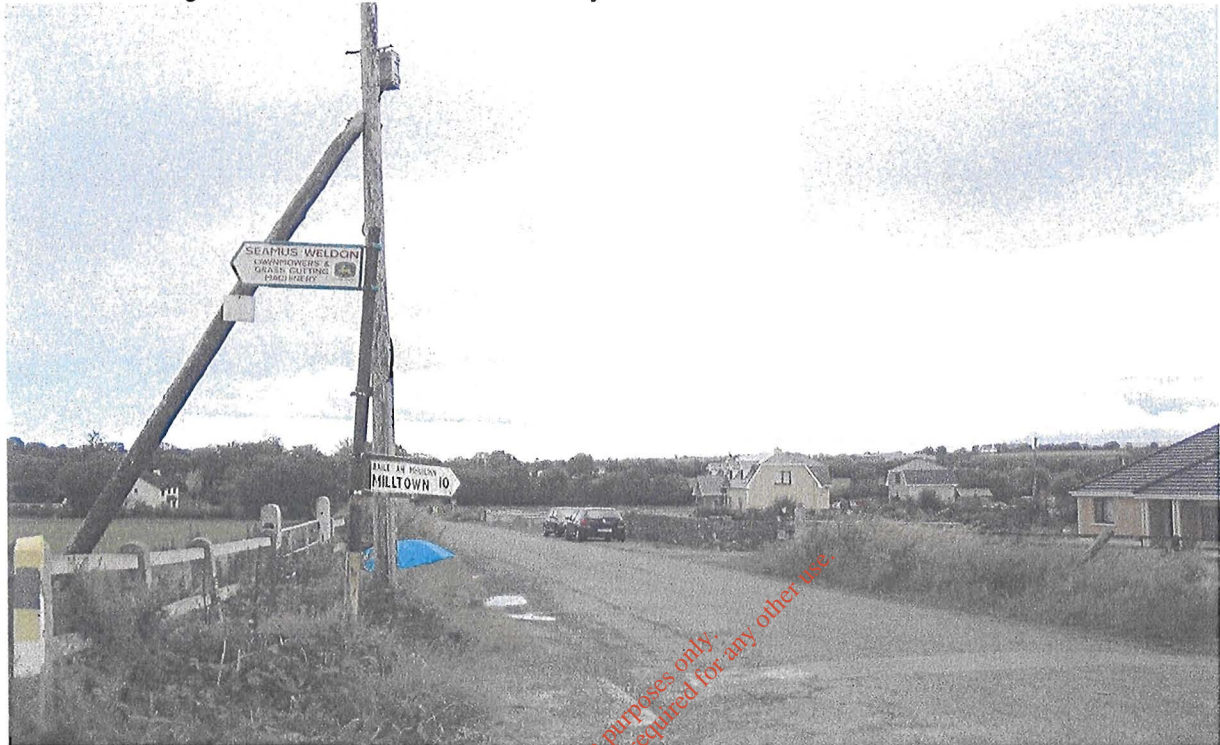
Figure 1.7 Ballyhar-Cleeny Road/Aghacurreen Road Junction, looking left
