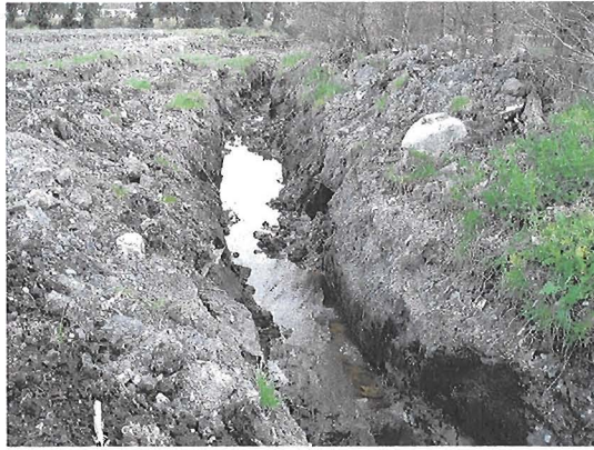
Recently excavated channel
