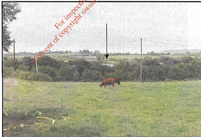
Plate 1.6 Looking northwards to the site, indicating the roof of the existing structure
