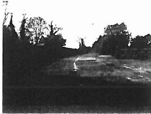
View Travelling West 200m from Current Entrance
