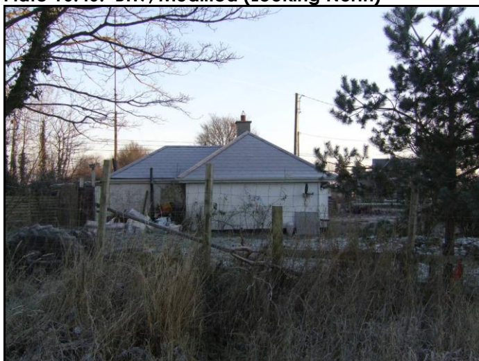
Plate 16.46: BH9, Modified (Looking North)
