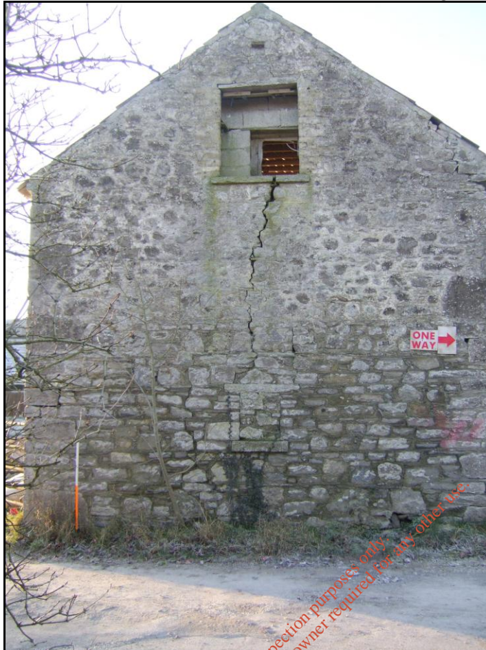
Plate 16.34: BH6, Northern Elevation of Outbuilding 2 (Looking South)
