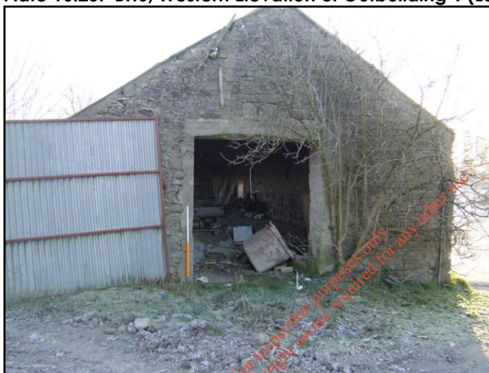
Plate 16.25: BH6, Western Elevation of Outbuilding 1 (Looking East)
