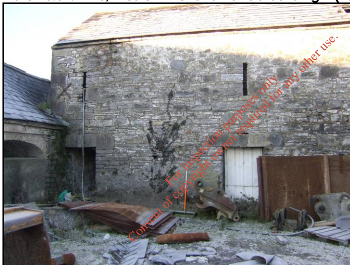
Plate 16.37: BH6, Western Elevation of Outbuilding 2 (Looking East)
