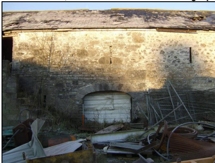
Plate 16.36: BH6, Western Elevation of Outbuilding 2 (Looking East)
