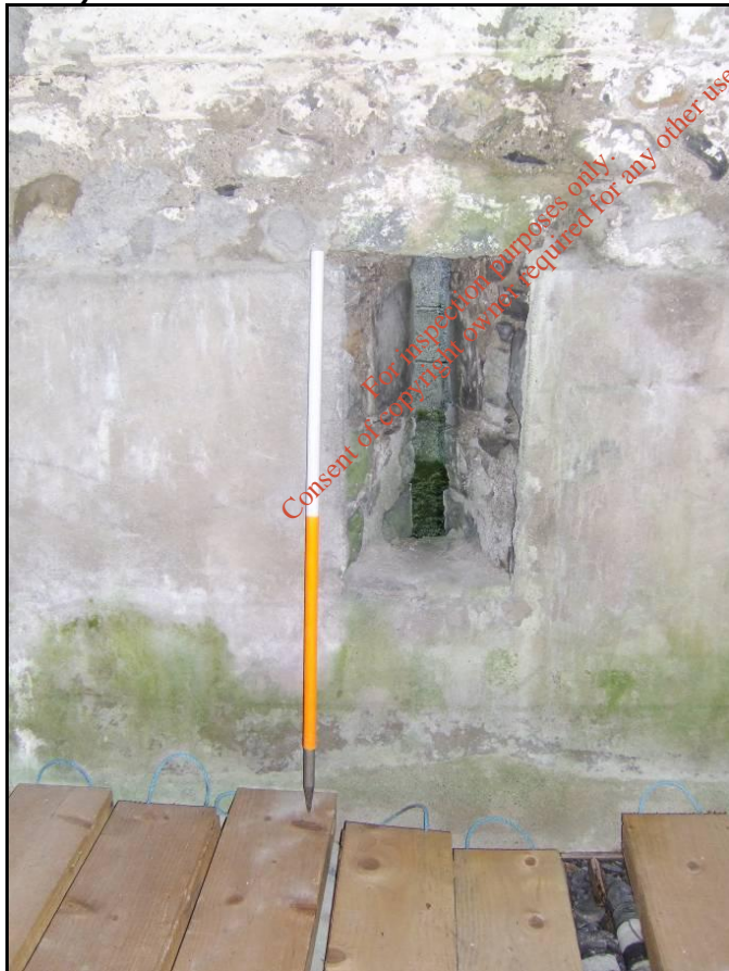
Plate 16.42: BH6, Interior of Outbuilding 3 showing Silt Window Ope (Looking North)
