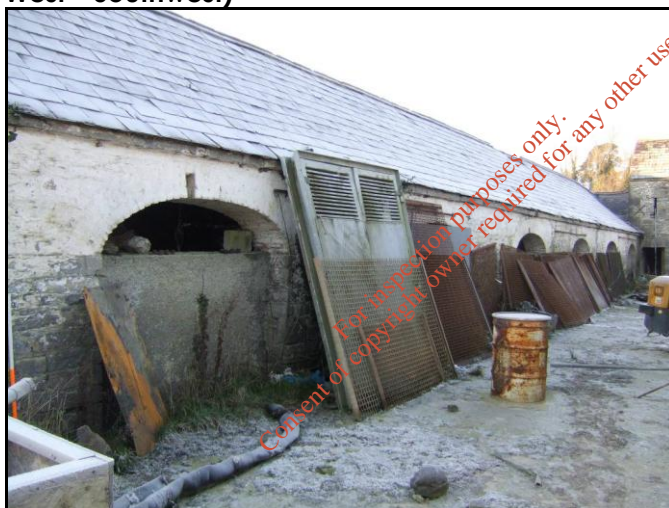
Plate 16.39: BH6, Northern Elevation of Outbuilding 3 showing Arches (Looking West – Southwest)
