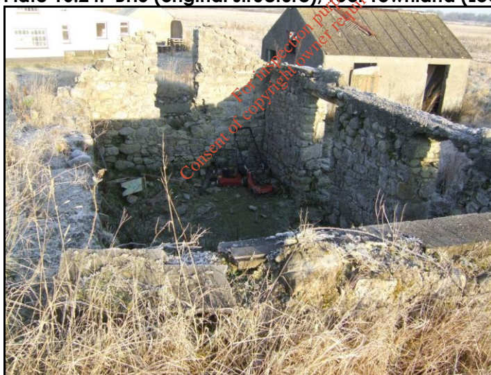
Plate 16.24: BH5 (original structure), Toor Townland (Looking South)
