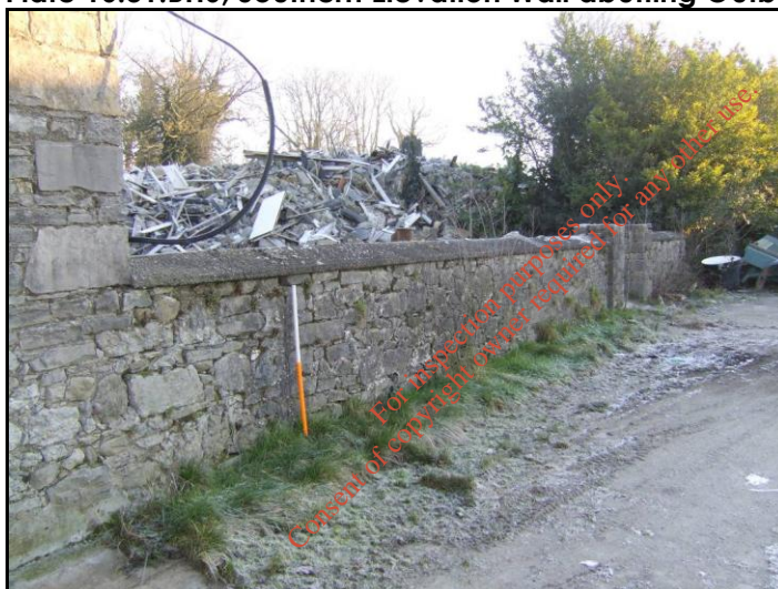
Plate 16.31: BH6, Southern Elevation Wall abutting Outbuilding 1 (Looking North)
