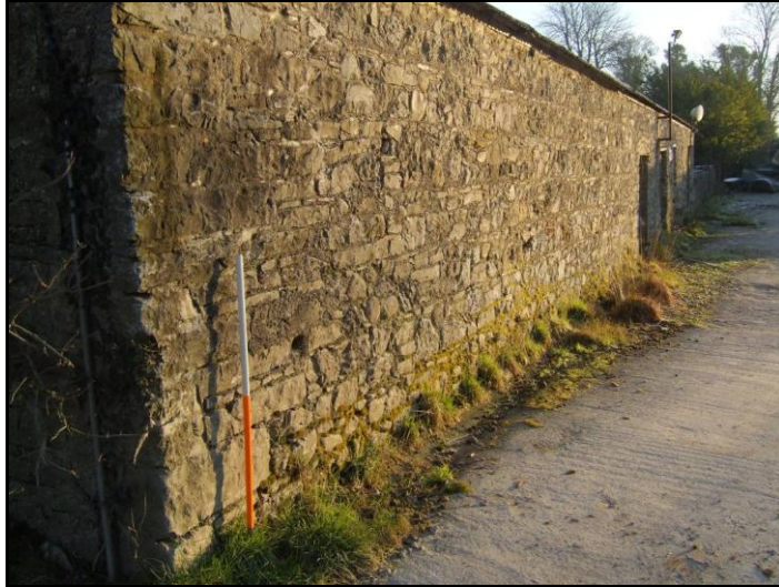
Plate 16.27: BH6, Southern Elevation of Outbuilding 1 (Looking Northeast)
