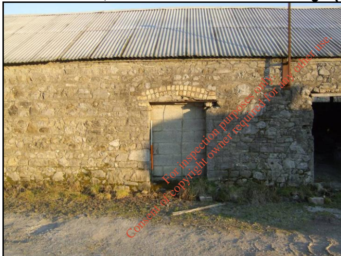
Plate 16.28: BH6, Southern Elevation of Outbuilding 1 (Looking North)
