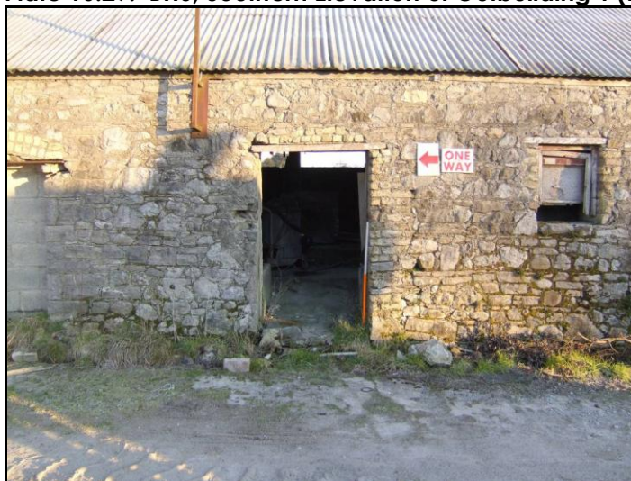
Plate 16.29: BH6, Southern Elevation of Outbuilding 1 (Looking North)
