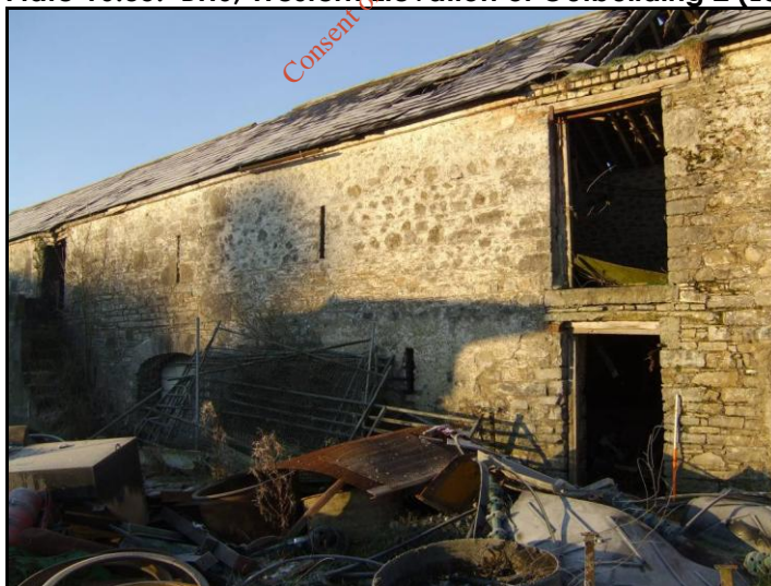
Plate 16.35: BH6, Western Elevation of Outbuilding 2 (Looking Southwest)
