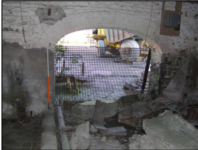
Plate 16.41: BH6, Interior of Outbuilding 3 (Looking North)
