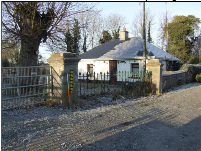
Plate 16.47: BH9, Modified Gatehouse (Looking Southwest)
