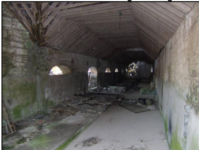
Plate 16.40: Interior of Outbuilding 3 showing Doorways (Looking East)
