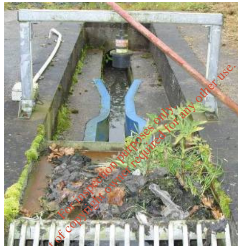
Photograph 1 Inlet Works
