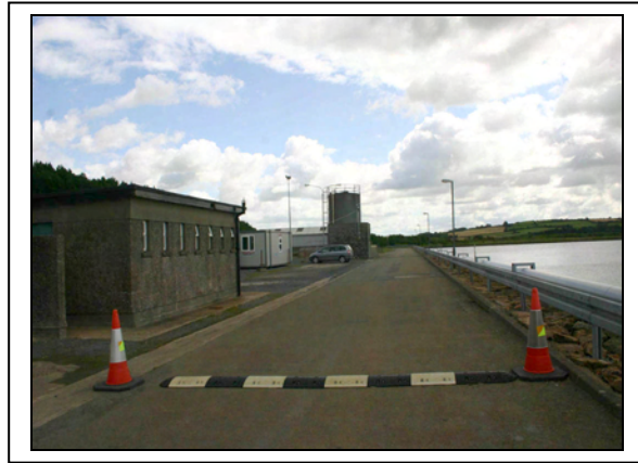
Plate 17.8 Proposed construction area, from W
