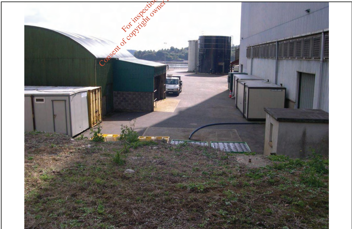
Location No: 28 Looking south from rear of main building.
