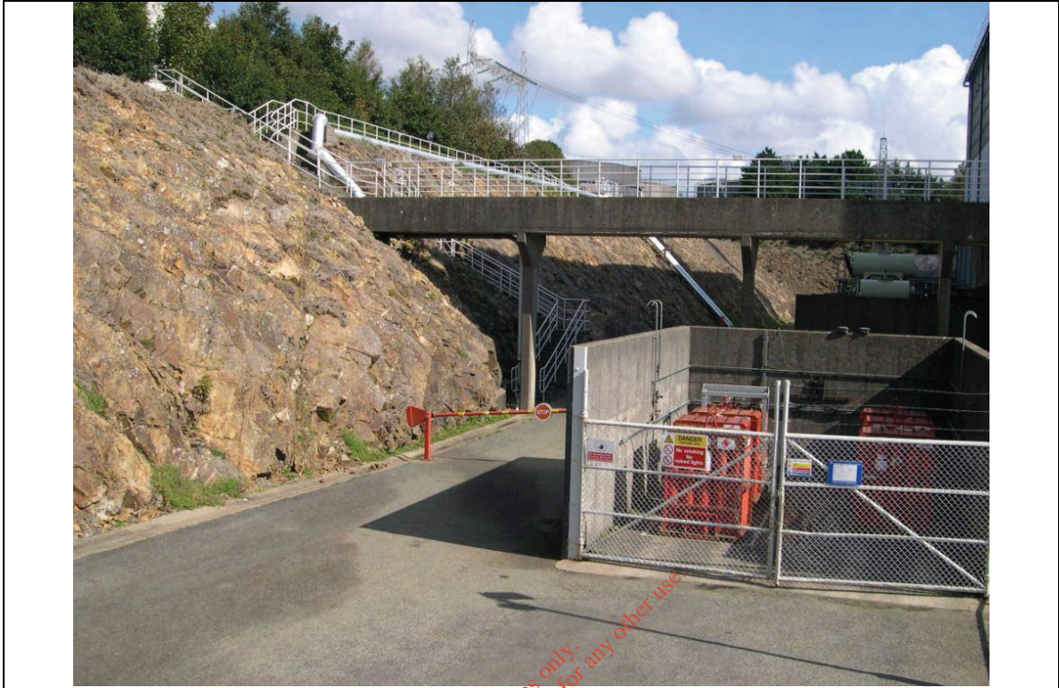
Location No: 25 View east at rear of main building.
