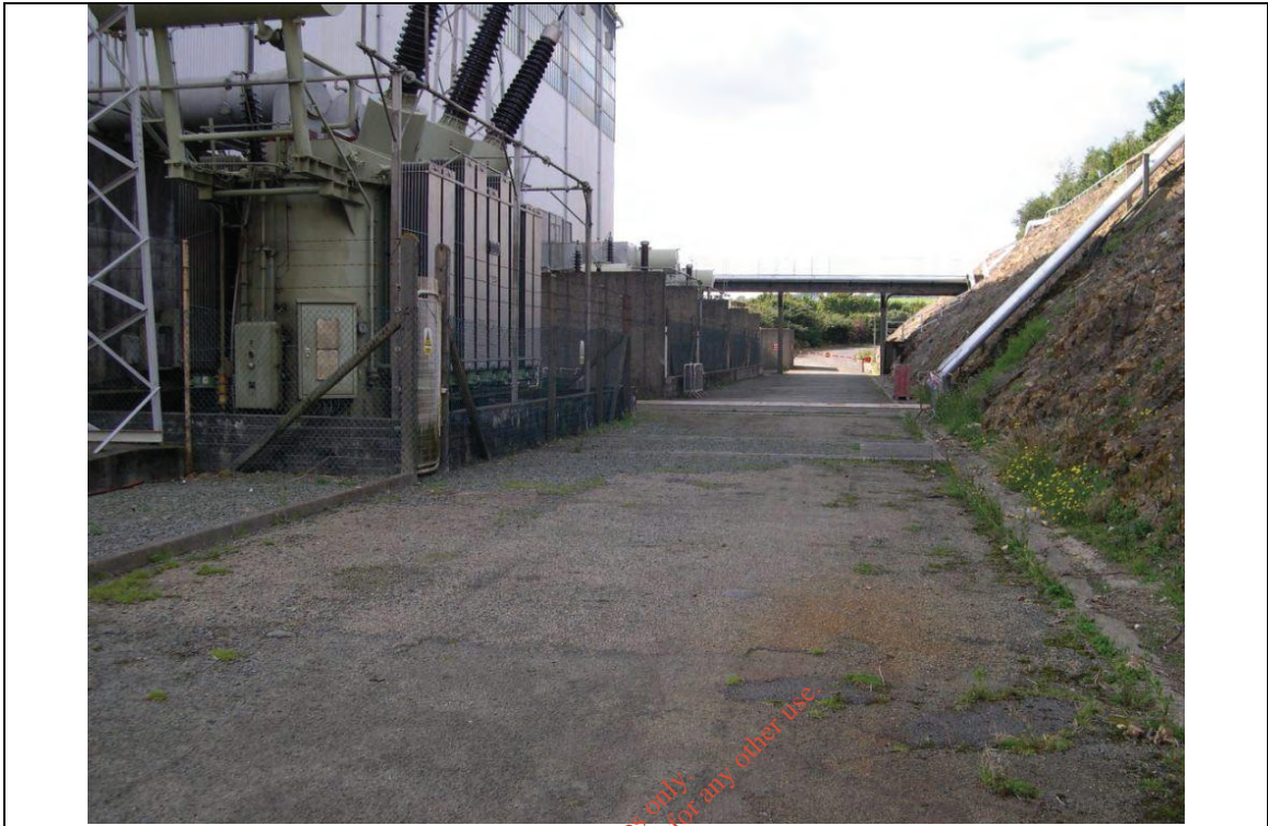
Location No: 27 View west at rear of main building.
