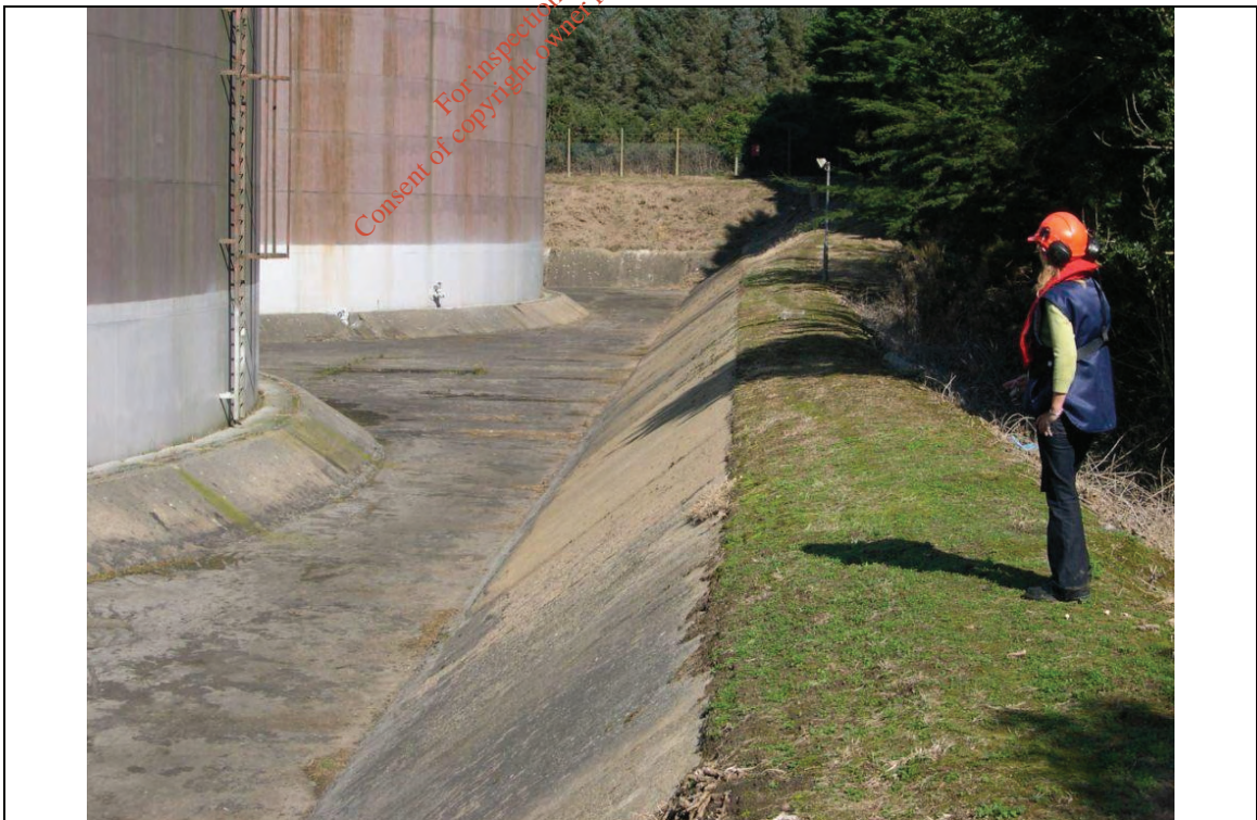
Location No: 21 View north along tank farm.
