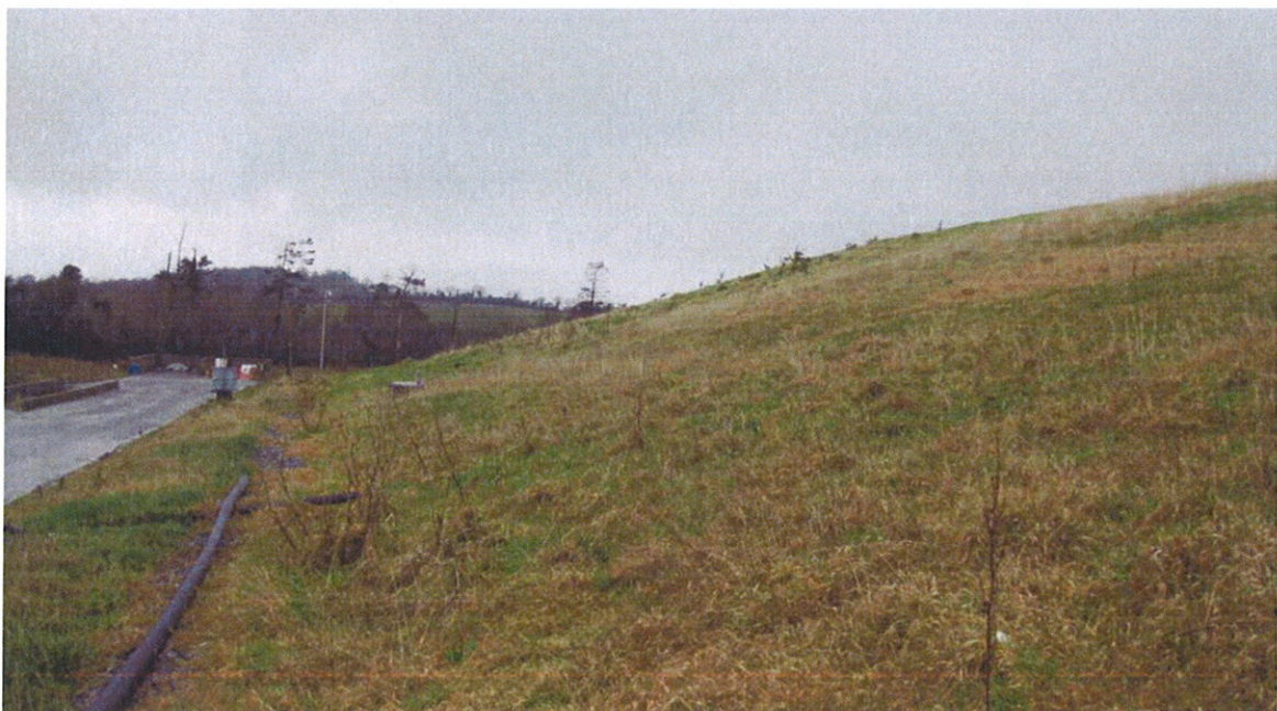
Photograph 2 Restored Slope to west of site
