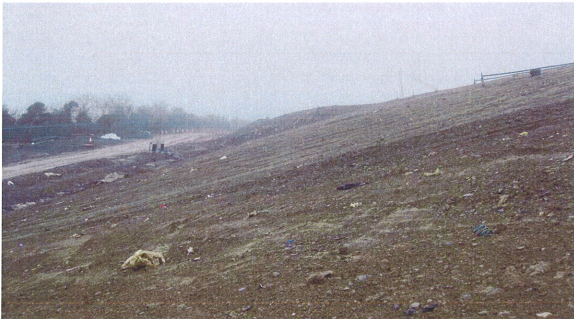
Photograph 5 Cell 3A south prepared for final capping
