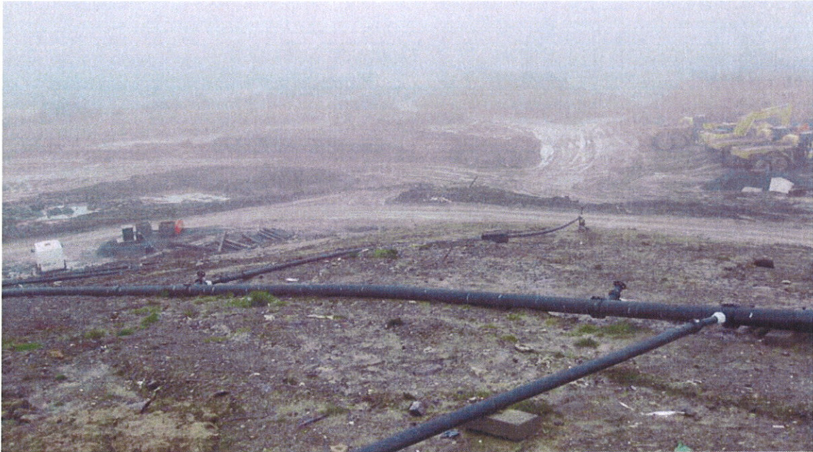
Photograph 4 Cell 3B east
