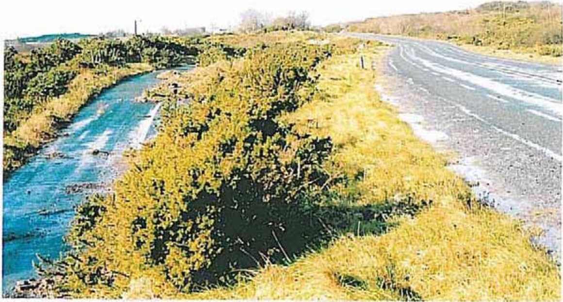
Plate 1. The section of the R311 from the landfill to Cartron is relatively recent, with remnants of the original road route still present. View is looking westwards, close to Derrinumeera.
