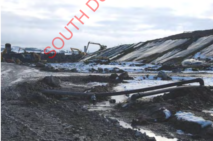
Plate 4: CoverTop 32 placed on side slopes of Cell 14.
