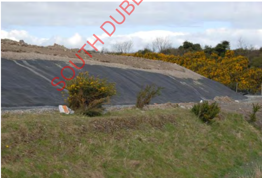
Plate 2: Partial capping material placed on side slopes at the rear of Cell 15. HDPE Liner welded to anchor trench.
