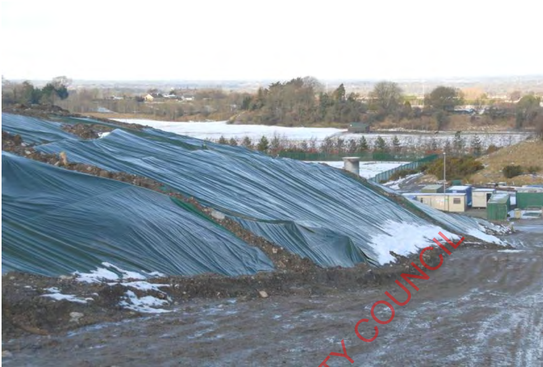
Plate 5: CoverTop 32 placed on side slopes of Cell 14 (Enclosed Flare in background)
