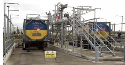
Figure 1.2.4 Picture of Tanker Loading/Unloading Bay
