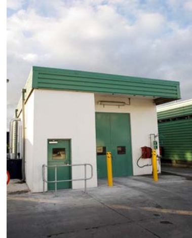
Figure 1.2.2 Picture of Repack Room
