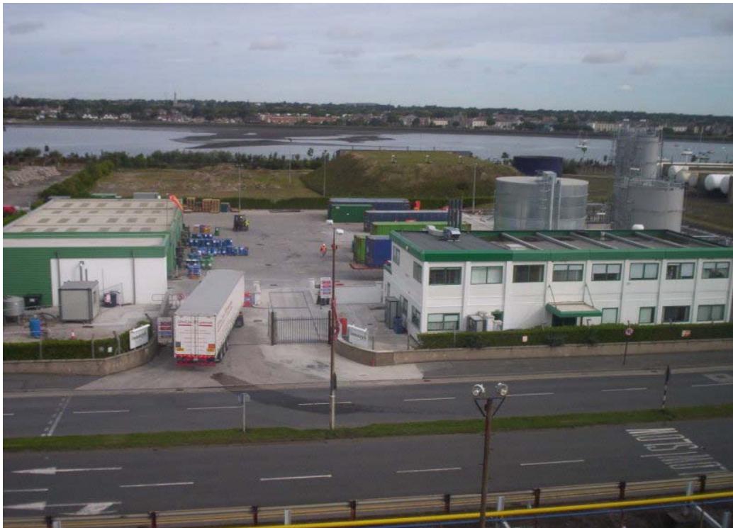
Figure 1.2.1 Picture of Dublin Port HazWaste Facility
