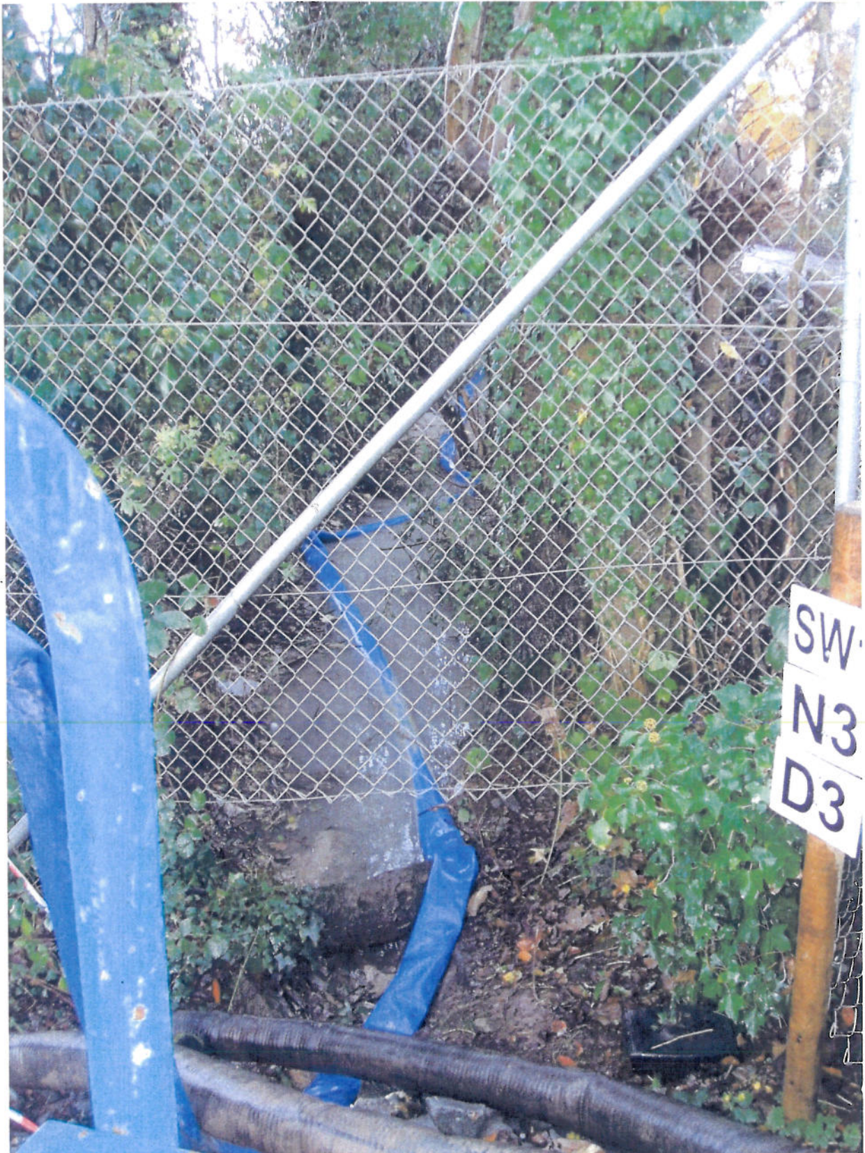
Photo No.1 View of drain at storm water discharge point SW1.
