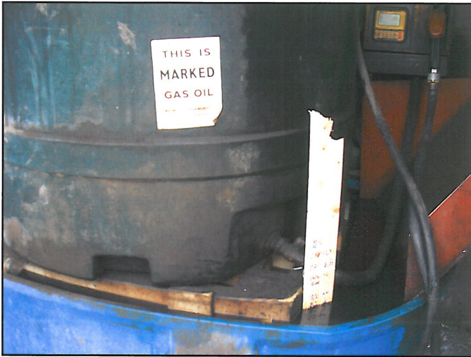
Photo ID: Diesel Bund 2 - Day 2 (03/11/2009)
