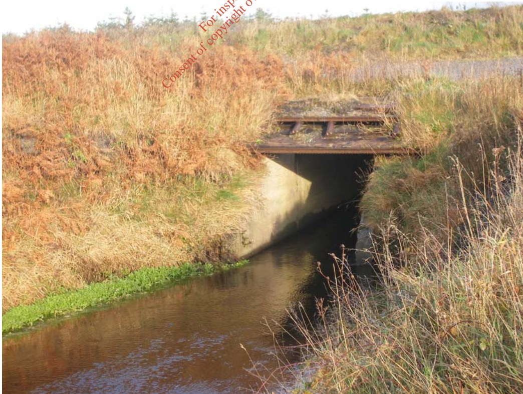
Figure 5-8 Structure 2, 2.5 km downstream upstream view -3300 mm box culvert
