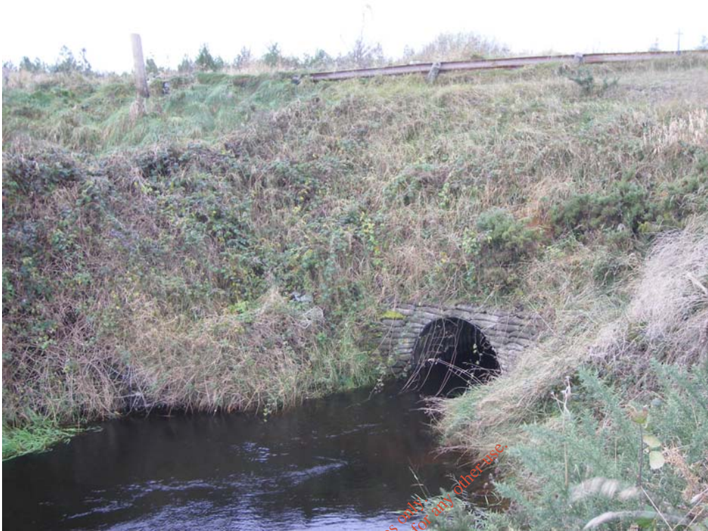
Figure 5-7 Structure 1, Mongagh Bridge (upstream view) – 3000mm culvert
