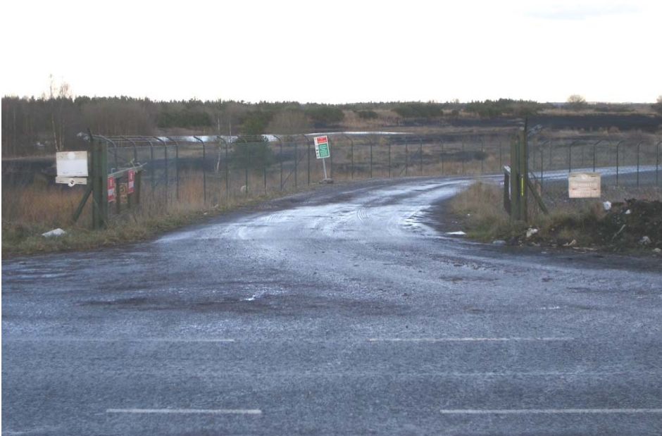
Figure 2-1 Existing entrance to site
