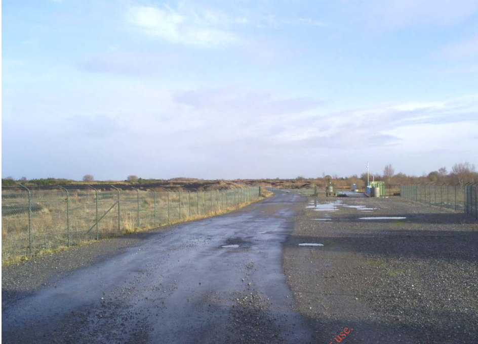
Figure 2-2 Existing weighbridge & haul road
