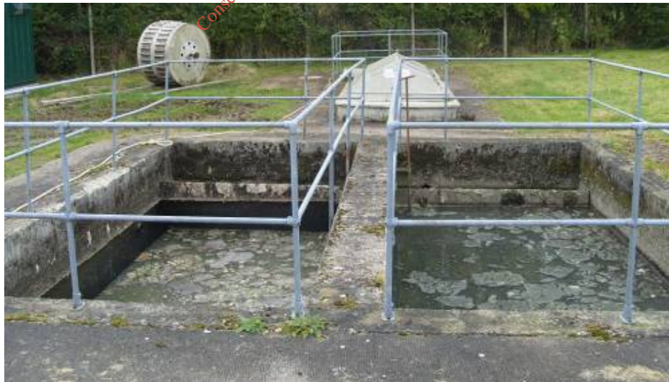
Photograph 2 Settlement Tanks
