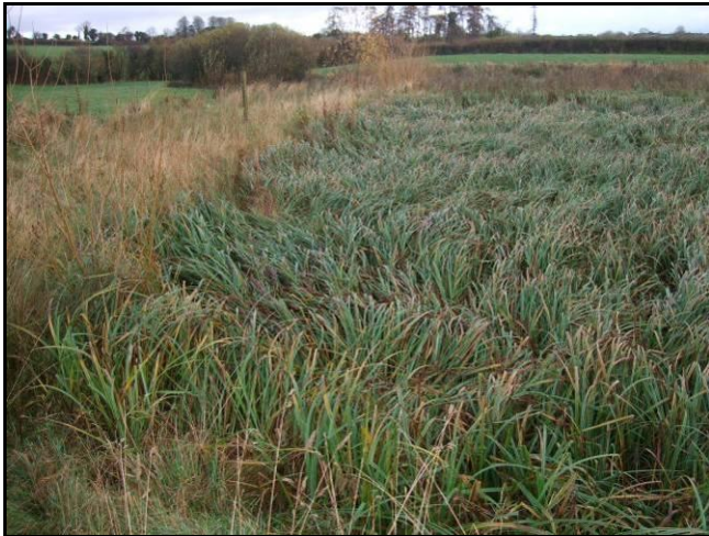
Plate 1 The Clogh WwTP has a primary and secondary treatment process, the latter is a well developed reed bed system as shown.
