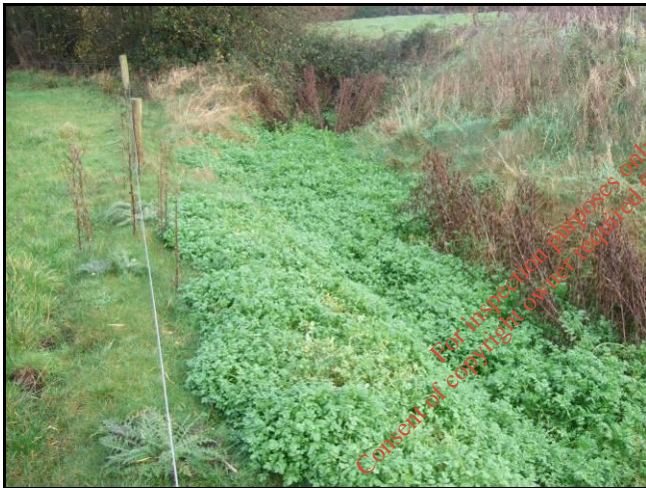
Plate 2 The back drain located to west of the reed beds which receives discharge from the latter.
