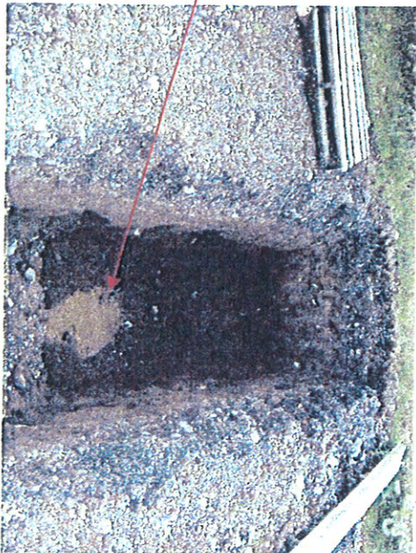
Trial Hole & Existing Building
