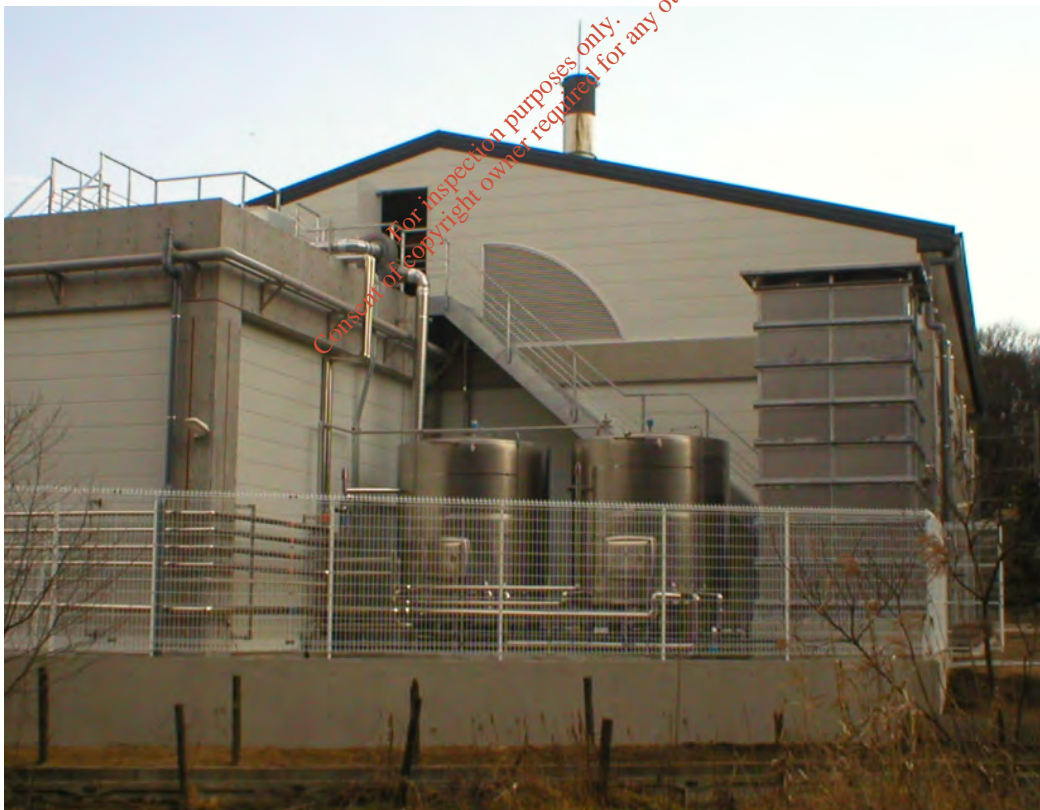
Fig. 10. Percolate storage at a Bioferm facility in Japan
