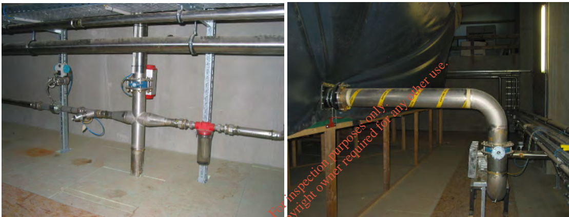
Fig. 13. The pneumatic gas collection system on the roof of the fermenters (left) and the gas transfer blower to the gas bag located in the roof space above the fermenters (right).
