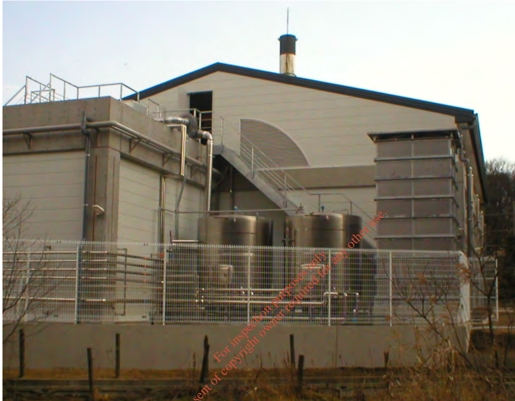
Fig. 9. Percolate storage at a Bioferm facility in Japan.
