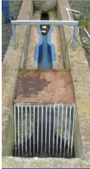
Photograph 1 Inlet Works
