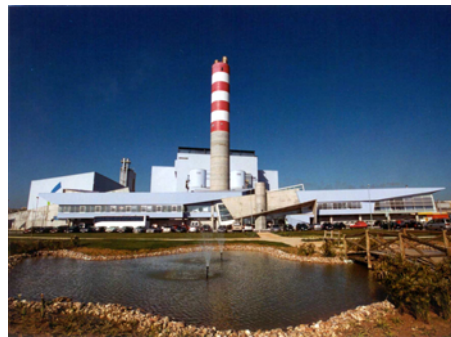
Incinerator in Portugal
