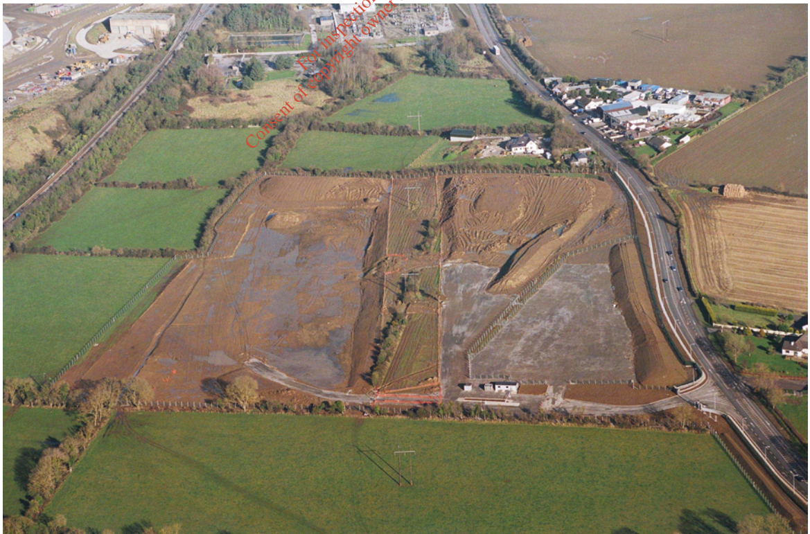
Figure 5.5 Overview of site development
