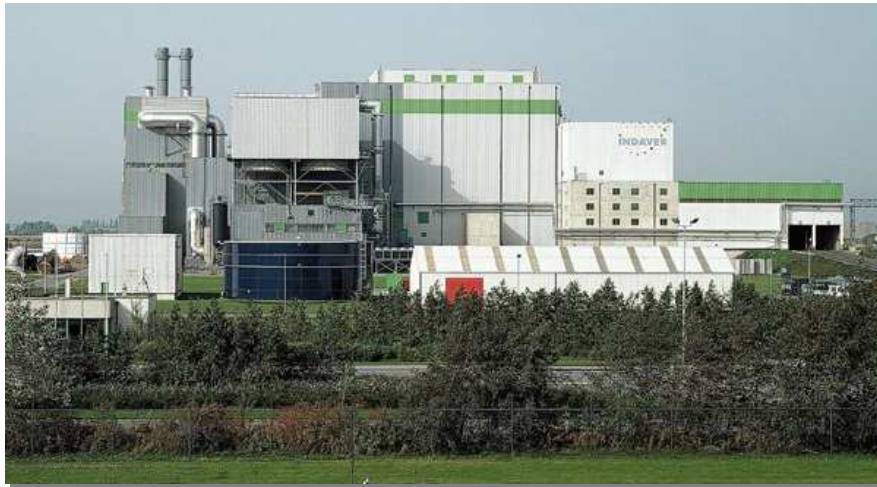
Figure A.1.b: Indaver NV facility in Flanders, Belgium
