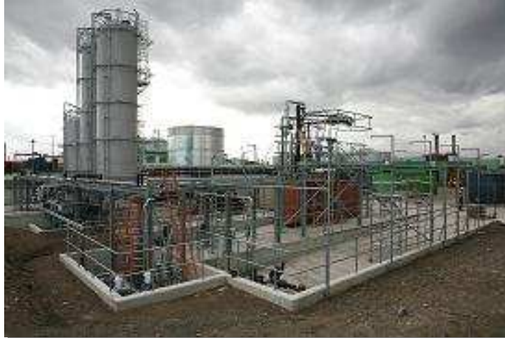
Figure A.1.c: Indaver Ireland Limited solvent blending facility in Dublin Port
