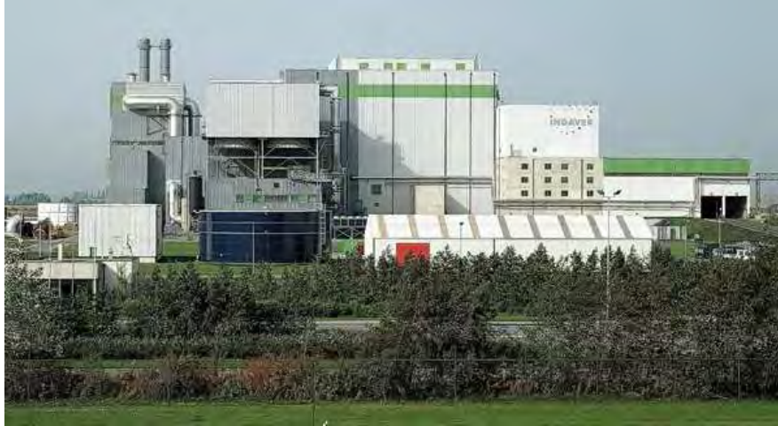
Figure 3. Municipal waste-to-energy facility, Flanders, Belgium
