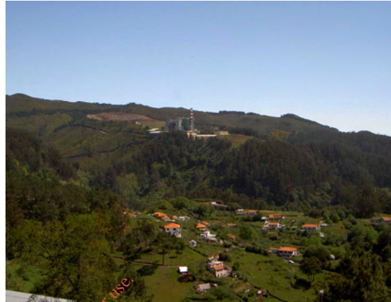
Waste-to-energy facility on Island of Madeira
