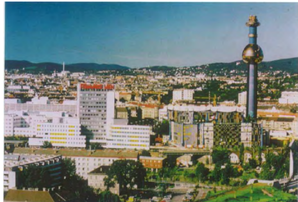
Waste-to-energy facility located in the centre of Vienna
