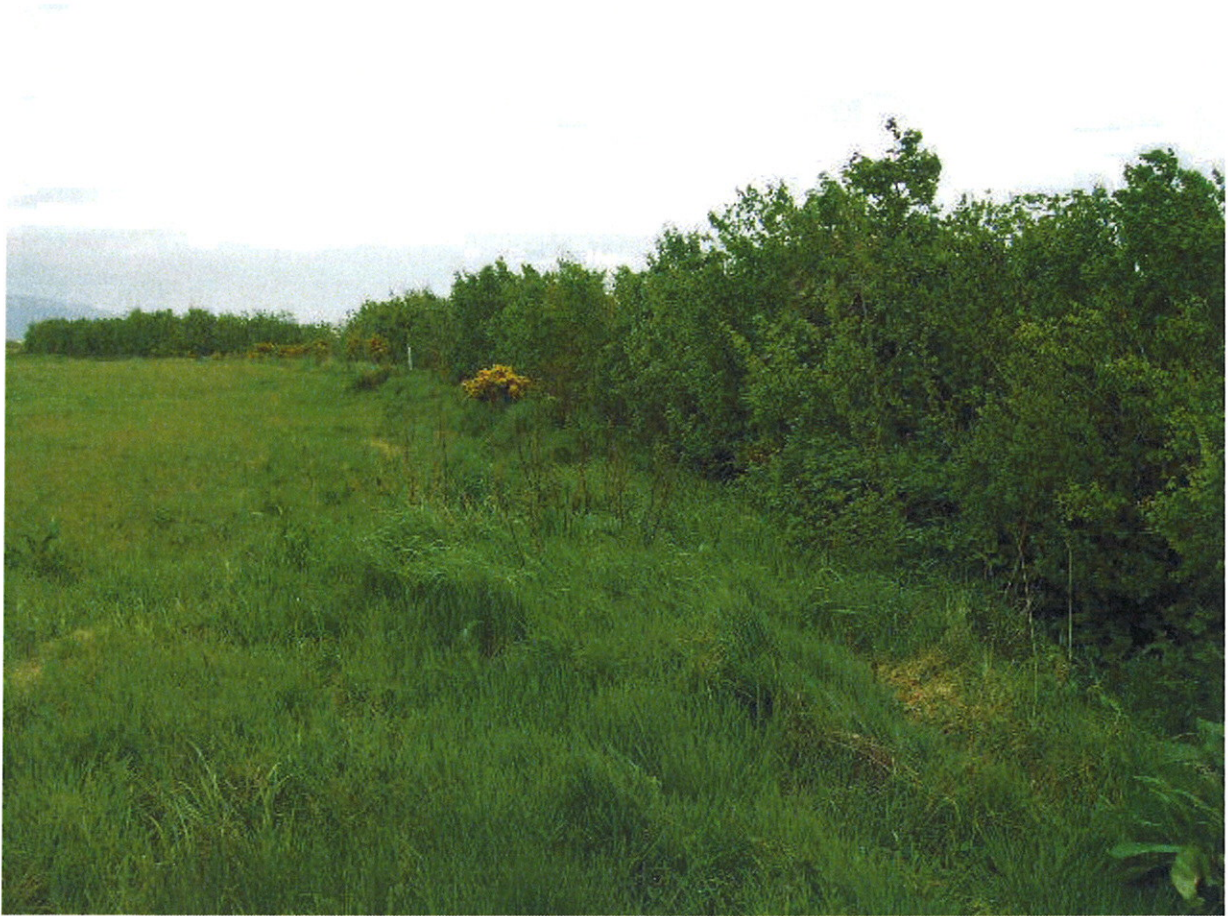
Photo 4: General view of Southern Slope (Top)
