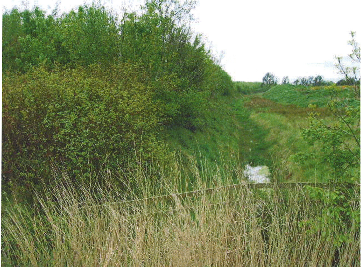
Photo 8: General view of Northern Side Slope (Toe)
