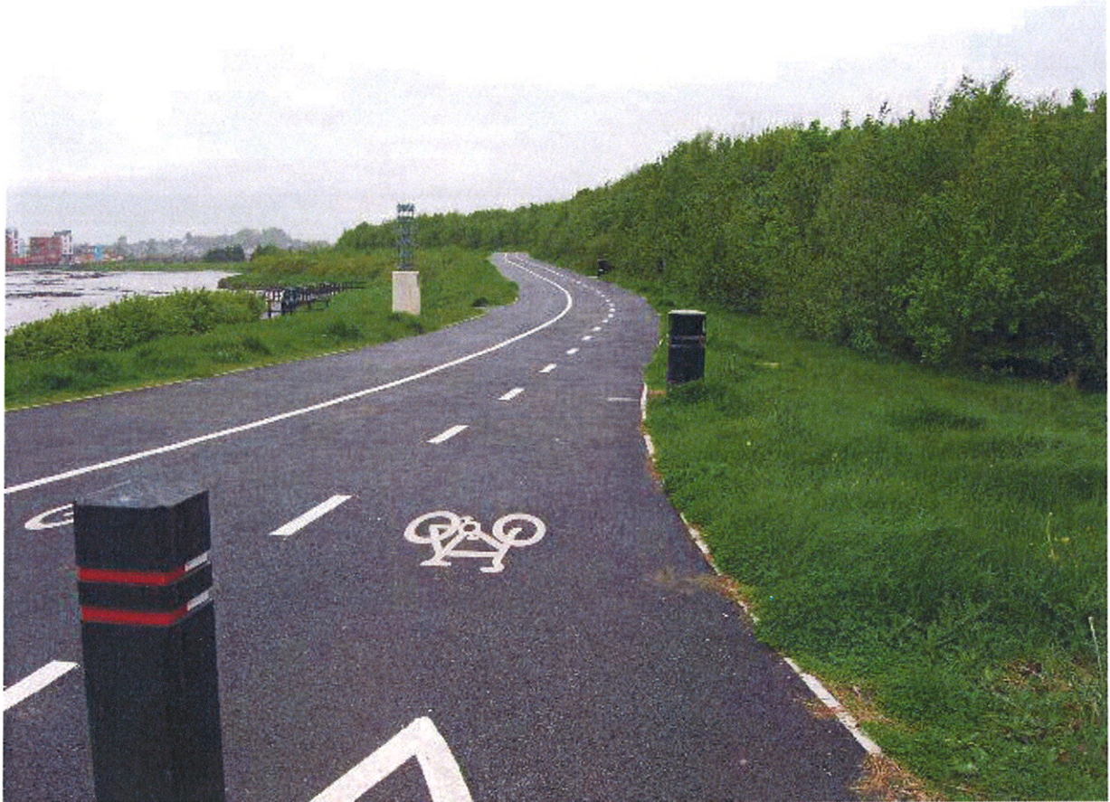
Photo 3:General view of Southern Slope (Toe)
