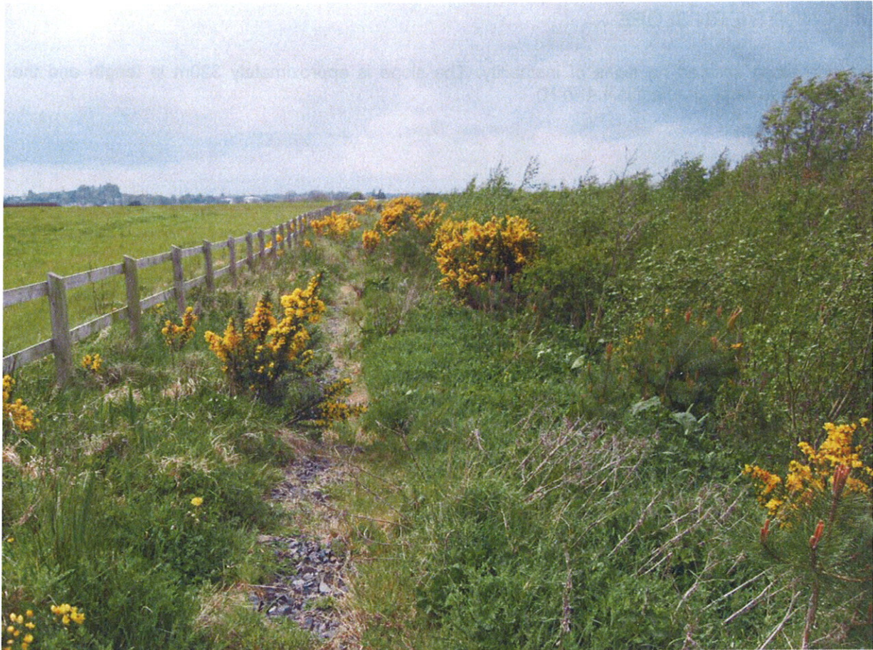
Photo 9: General view of Northern Side Slope (Top)
