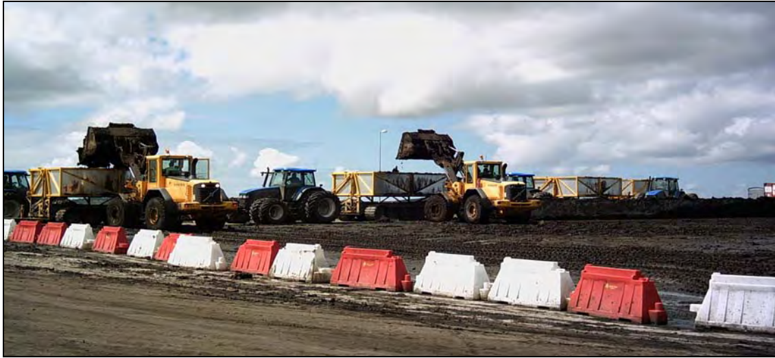
Plate 1: Loading of Haku Trailers from the Peat Reception Hardstand (as part of the previous peat deposition operation on site, 2005 & 2007)
