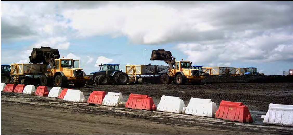
Plate 1: Loading of Haku Trailers from the Peat Reception Hardstand (as part of the previous peat deposition operation on site, 2005 & 2007)
