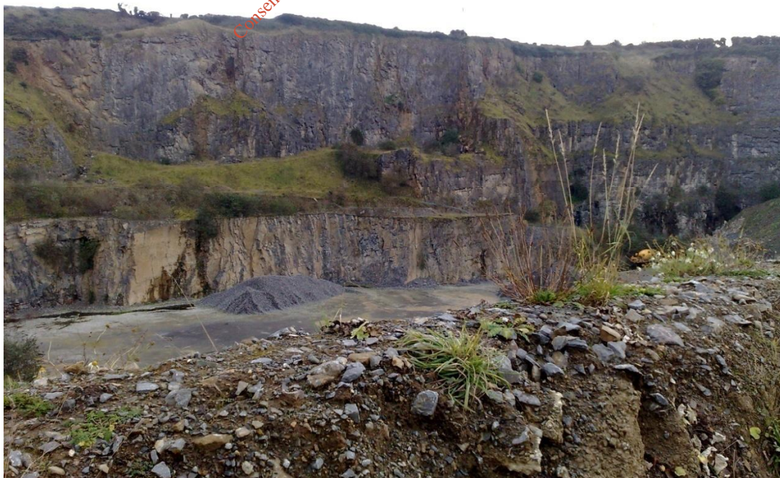
Plate 9.2 View of Quarry Area to be backfilled with Inert Soil
