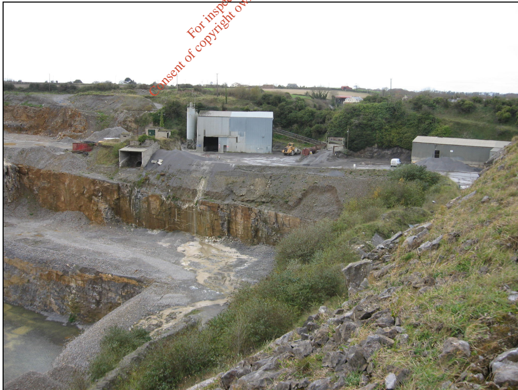
PLATE 6.2 Groundwater inflows at the northeastern quarry face
