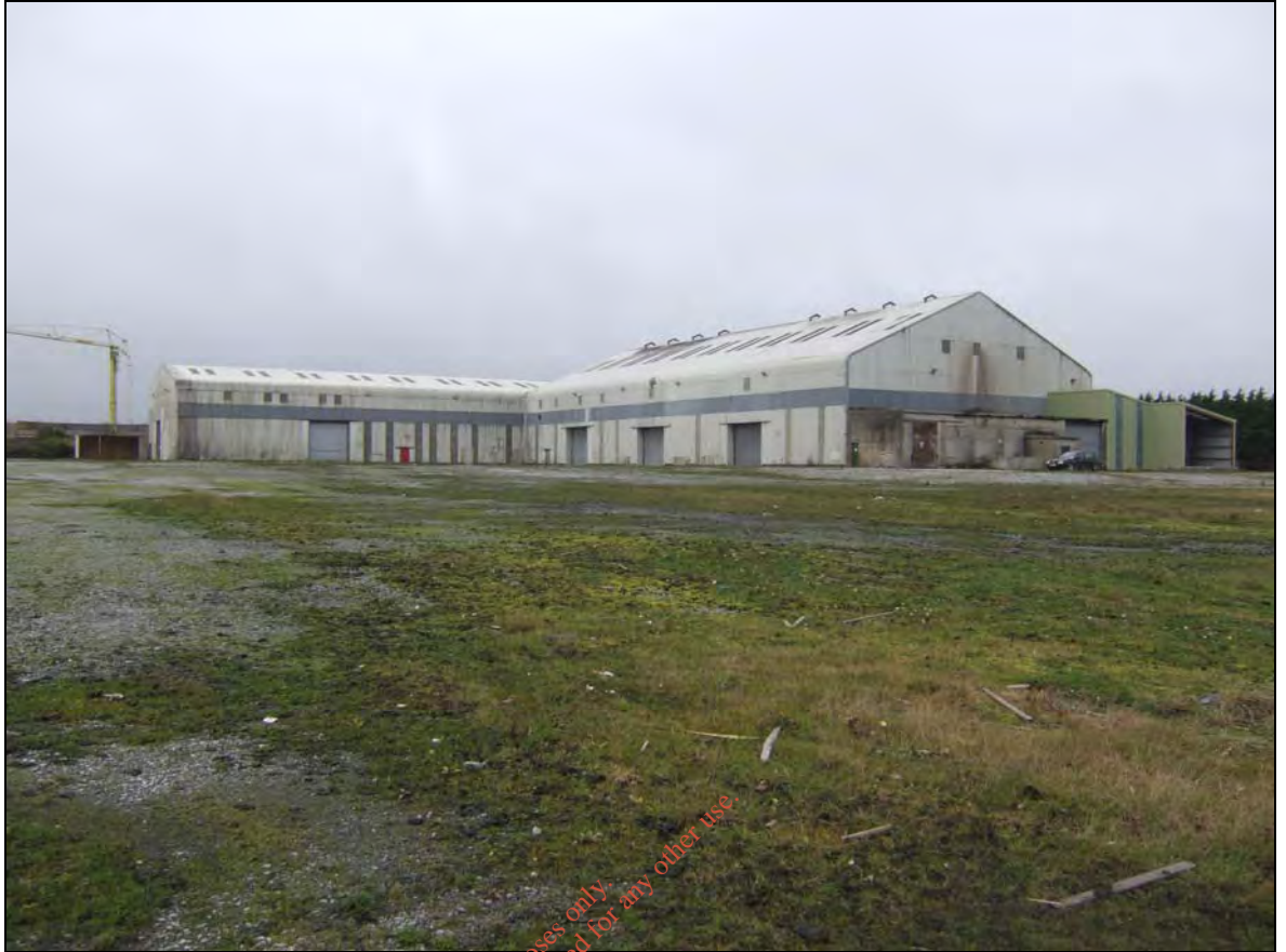
Plate 2.1 View of existing warehouse from the centre of the propose development site
