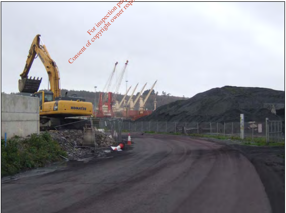
Plate 9.14 View along internal roadway within the Shannon Foynes Port Area
