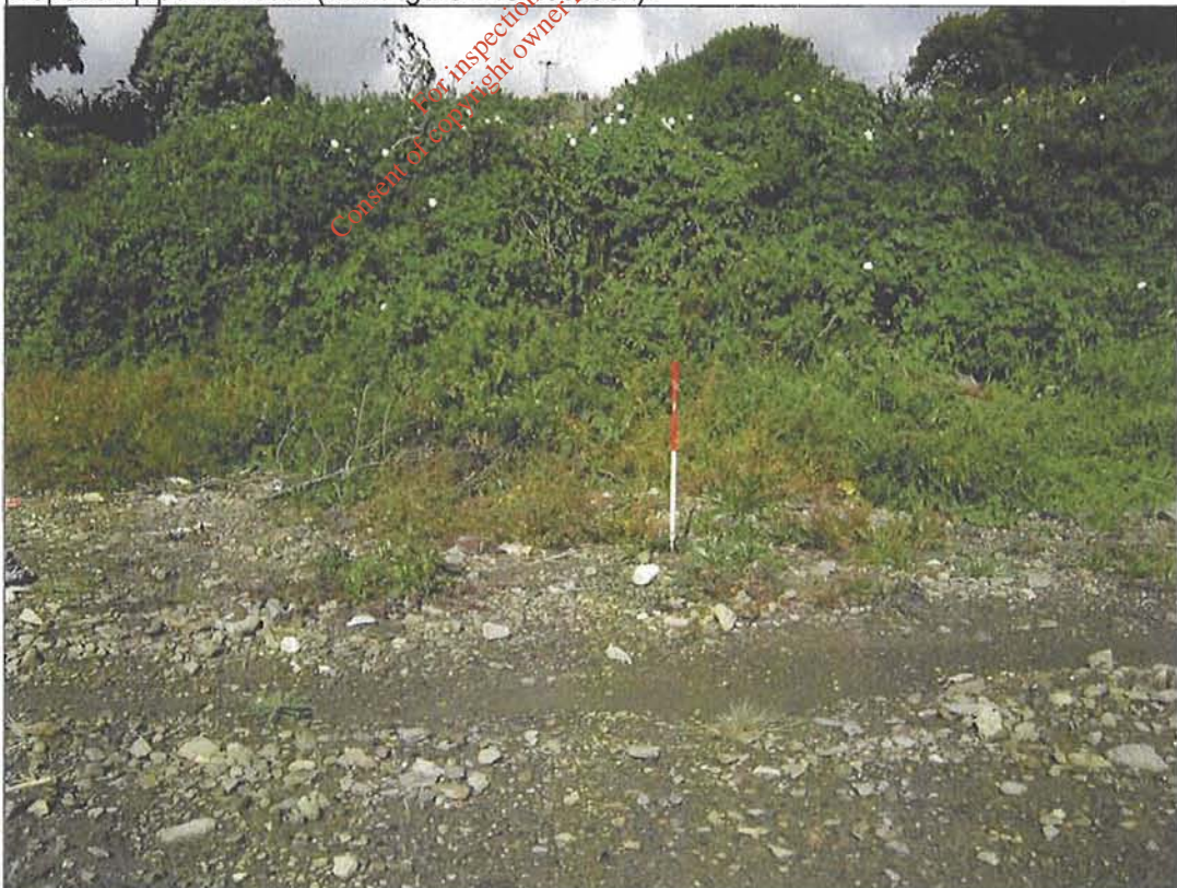
Plate 14: North-facing view of upper foreshore c.800m along pipeline route (see Figure 6 for location); 1m scale.
