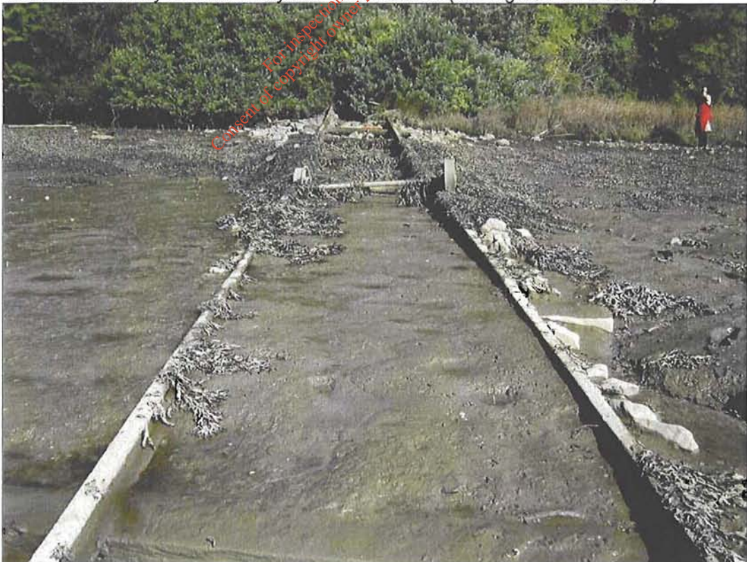
Plate 28: North-facing view of iron-trackway for boat-trolley/ launch located c. c. 1520m along proposed pipeline route (see Figure 7 for location); 1m scale.
