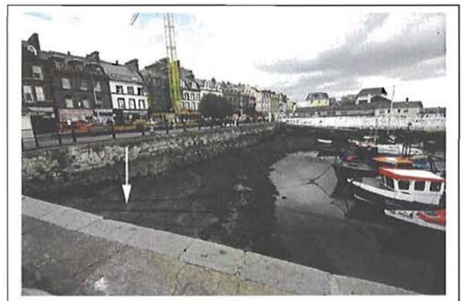
Plate 3.45. Proposed location of major pumping station at West Beach Cobh, viewed from southwest
