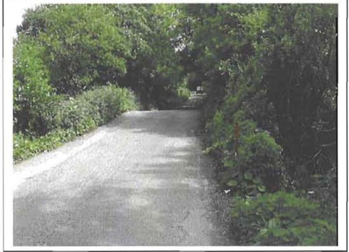
Plate 3.12. View southward over 'Dandy bridge' in Kilnagarry
