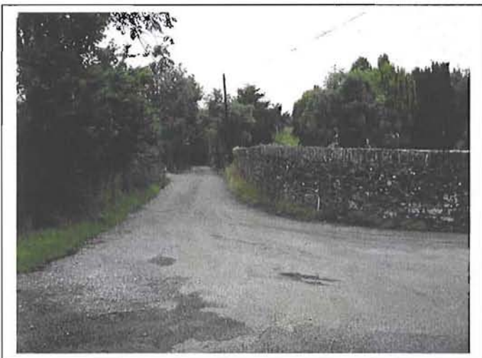
Plate 3.33. Route of pipe west of Clonmel church graveyard wall, from south
