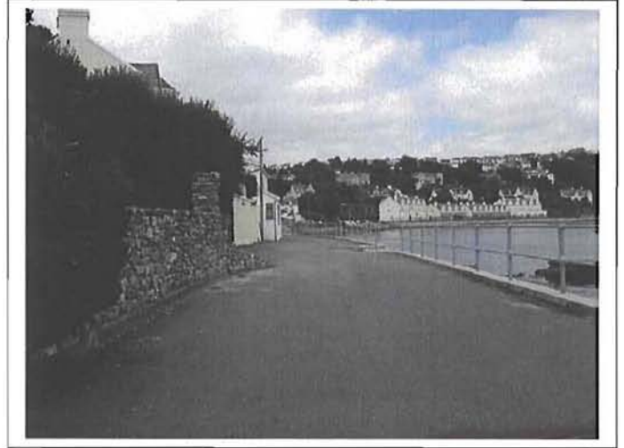
Plate 3.41. Pipeline route along roadway in White Point, from south
