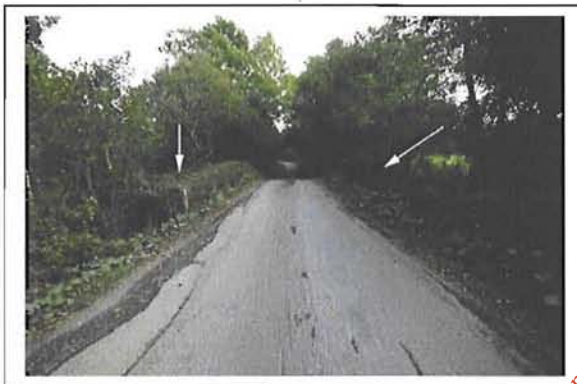
Plate 3.48. View of The Dandy Bridge (CH24), parapets arrowed, from west
