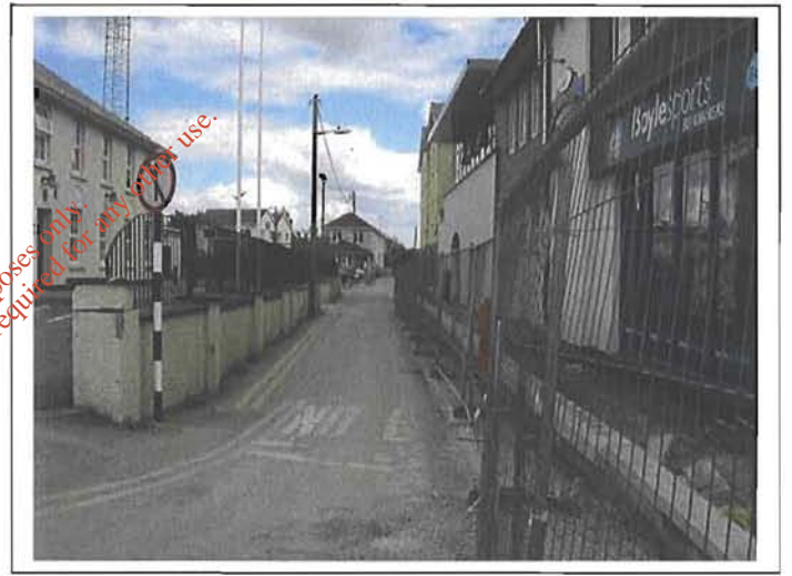
Plate 3.8. Pipeline route in the Carrigaline area, north of CH6, from west
