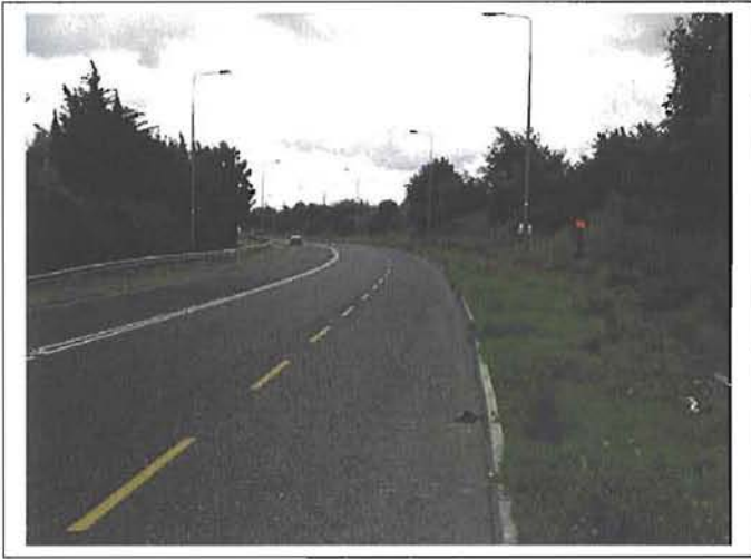
Plate 3.24. Pipe route along N28, from northwest
