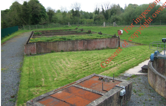
Sludge Drying Beds
