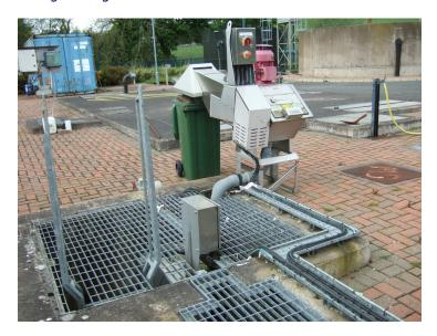
Overflow liquid is discharge by gravity to the storm water holding tank
