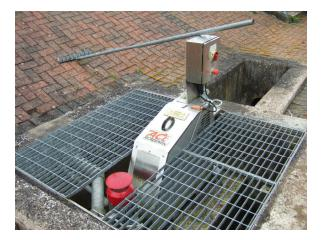
Overflow liquid is discharge by gravity to the storm water holding tank
