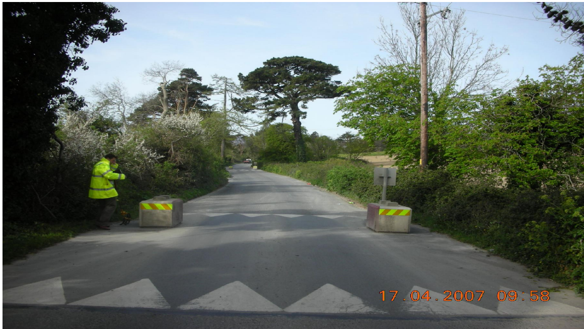
Plate 12.1 Existing road hump and road narrowing on Fassaroe Avenue
