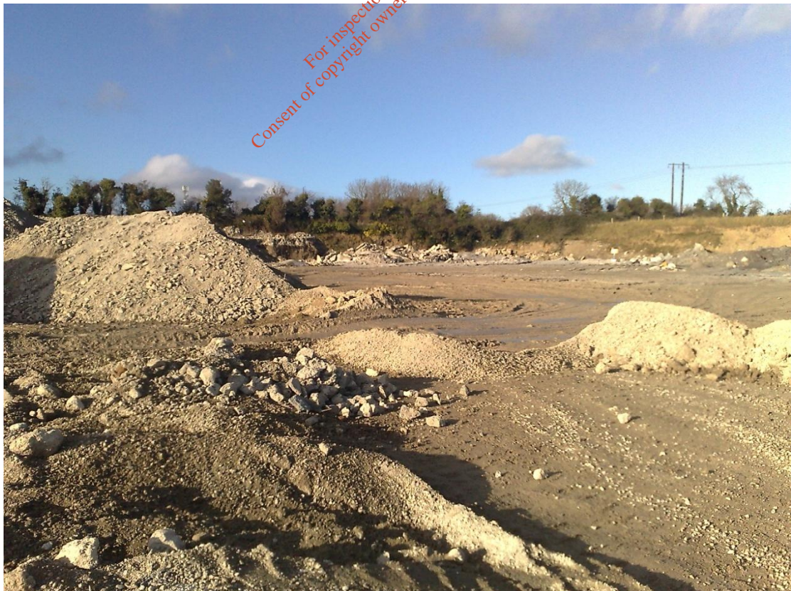
Plate 9.2 Construction and Demolition Waste Recovery Area
