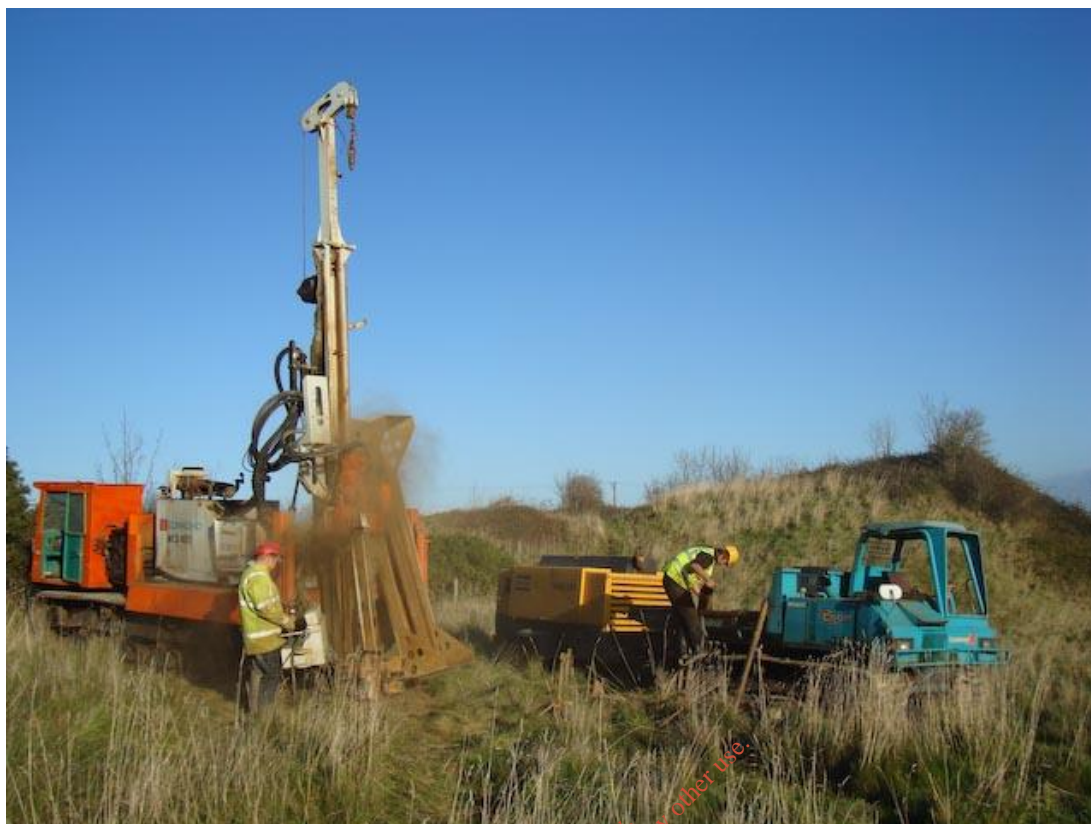
PLATE 6.3 Installation of Groundwater Monitoring Well BH1
