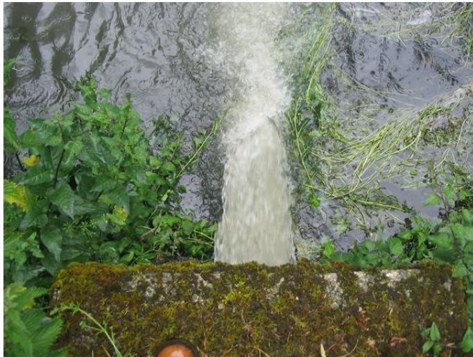
Fig 2 Outfall from Quarry Rd Pumping Station. (Existing)
