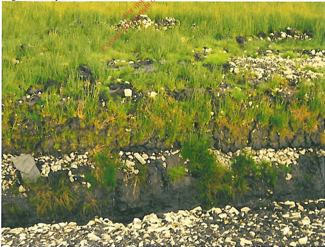
Condition of deposited Peat
