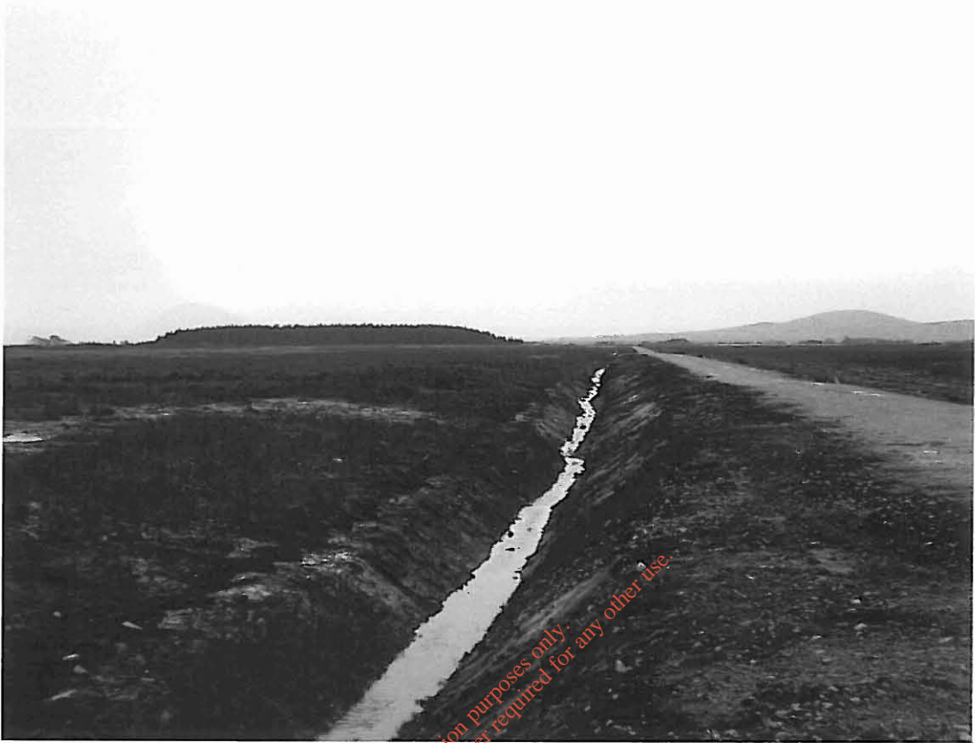
Bay 4 North Drain
