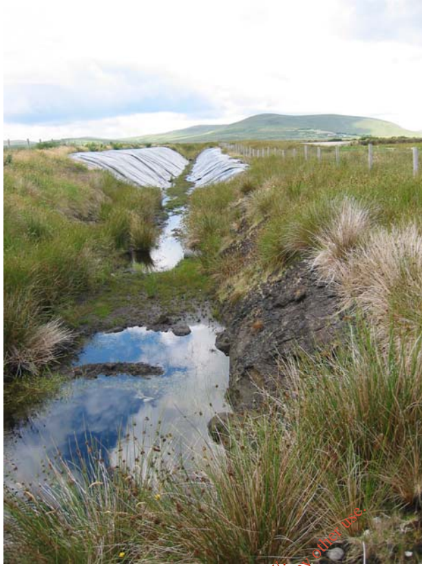
Plate 6.18 Lined drain at the southern end of the site
