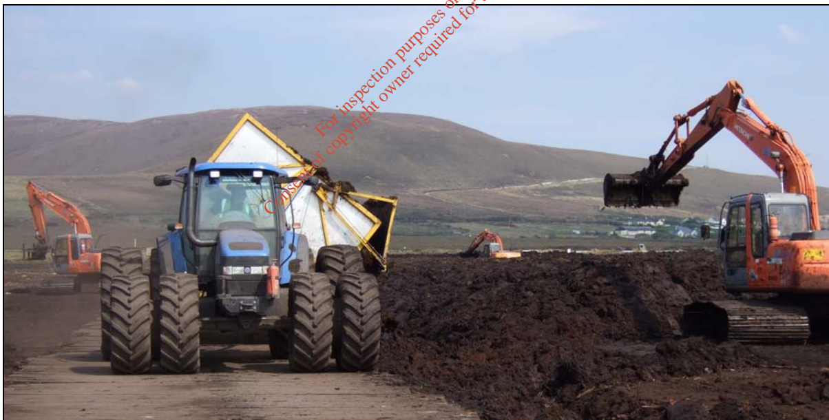
Plate 2: Peat unloading from Haku trailers onto deposition area (as part of the previous peat deposition operation on site, 2005 & 2007)
