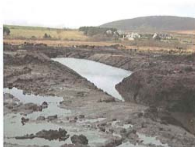
Plate 3 Water settlement pond 5 from west.
