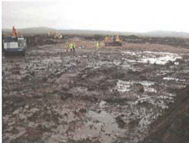
Plate 4 Administration area from north-east.
