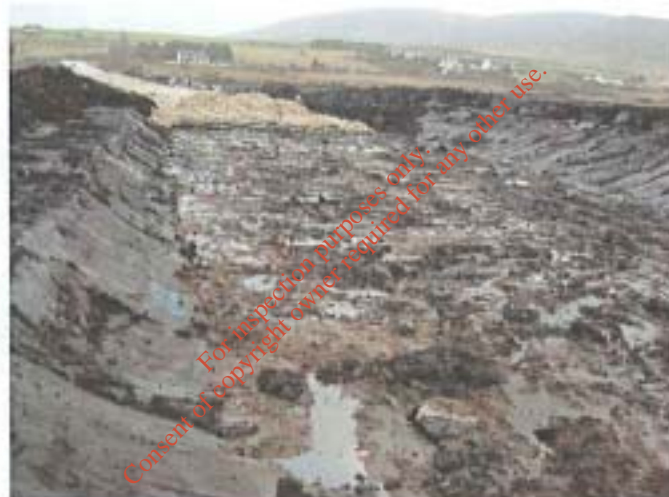
Plate 2 Site access road from south-west.
