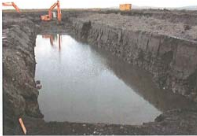
Plate 1 Water settlement pond 2 from north-east.
